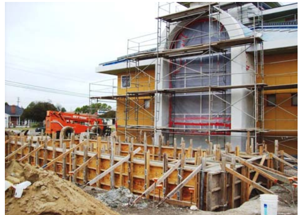
Irrigation Planter Development in front of the Library
