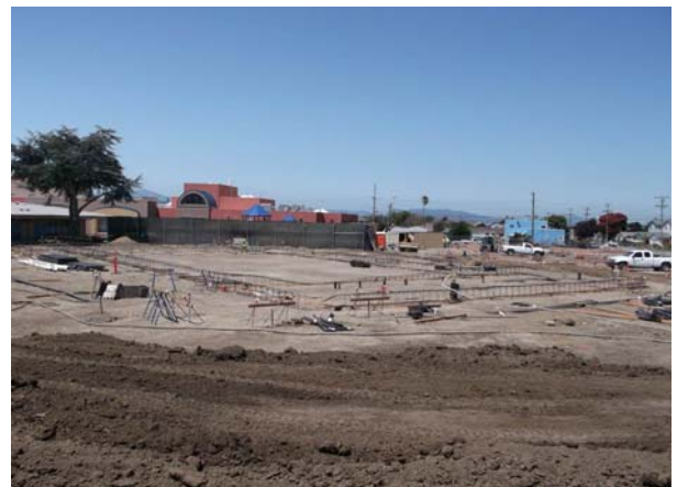
East Side of Site- Building C
