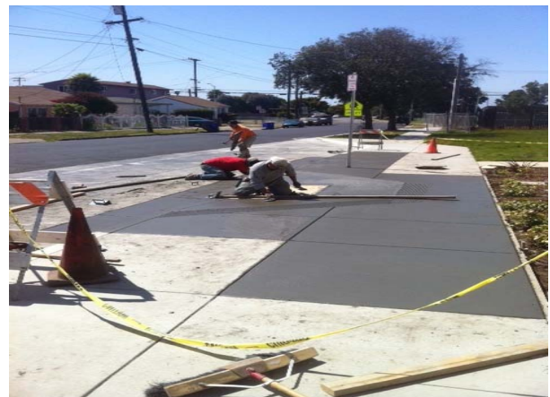
New AC Paving at 41st Street
