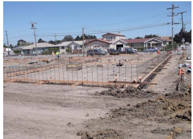
North Side of Site-Building B
