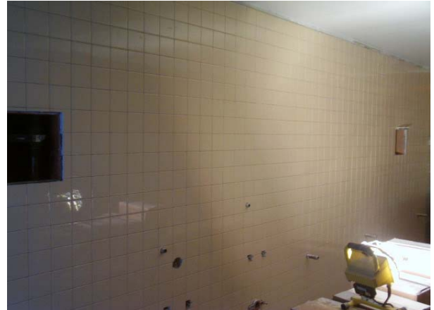
Stewart C122 Tile Install (Westward Wall)
