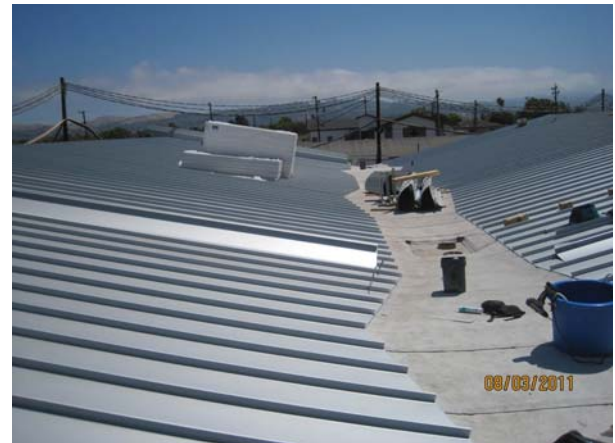
Roof Metal Panels
