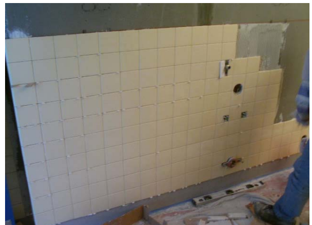
Stewart C137 Tile Install (Westward Wall)
