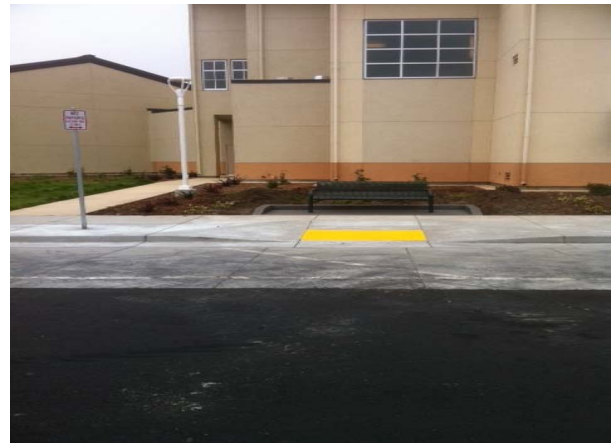
Accessible Ramp at 41st Ave.
