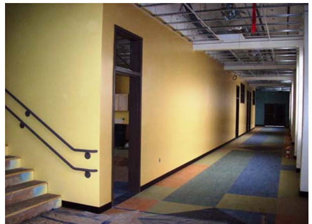
Area A, West Corridor - Finish Construction Progresses
