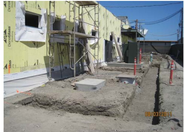
Footing for Trash & Electrical Enclosure
