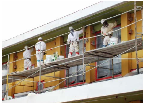
Stucco Exterior Advances Well - Final Color Coat Underway
