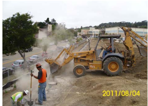
Retaining wall at Ashbury Ave drain rock backfill
