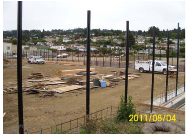
View from new tennis court fence post installed
