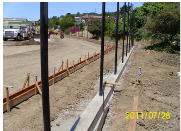
Mow band forming and fence post curb poured.
