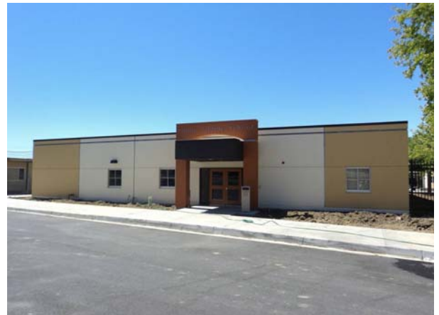
Front elevation of administration Building
