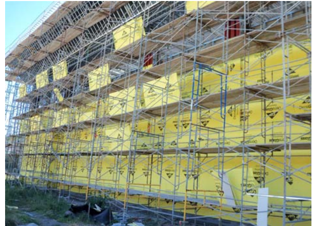
Building 8: Install Exterior Sheathing
