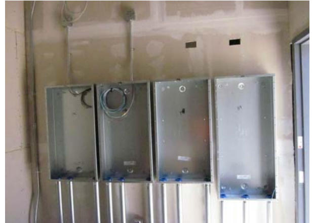
Building 9: Install Wall Insulation & Drywall
