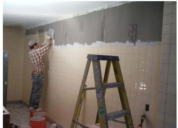
Stewart C123 Tile Install (Eastward Wall)
