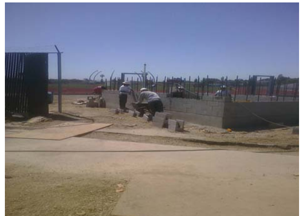
Concession Stand - CMU Block Erection
