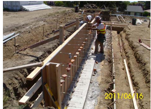
New tennis court retaining wall for new handicap ramp and stair
