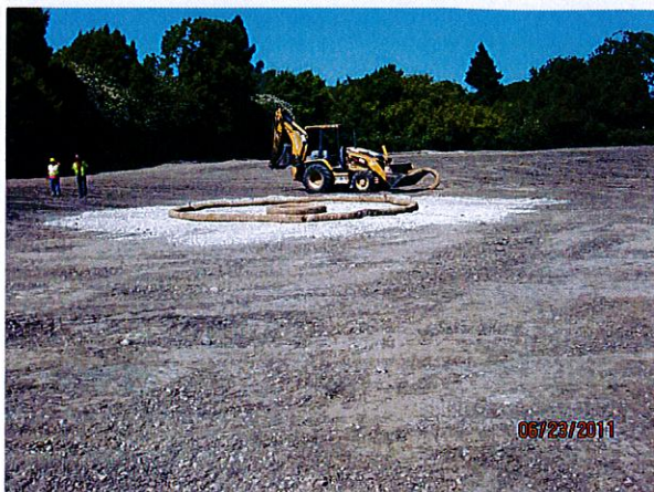
Installing the drain inlet protection
