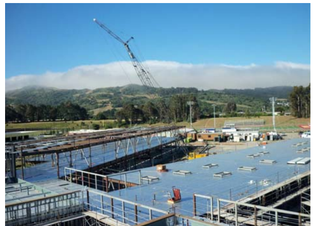
Building 6 & 7: Install Metal Roof Deck
