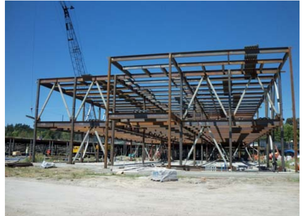
Building 7: Install Structural Steel
