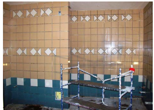
Bathroom Tile Finishes are Well Advanced
