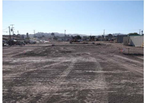
West Side of Site-Bldg. B & C Pad-COMPLETED
