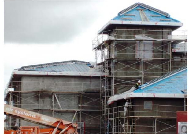
Stucco and Roof Construction Proceeds Well
