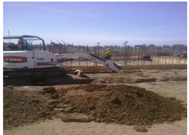
Sanitary Sewer Trenching
