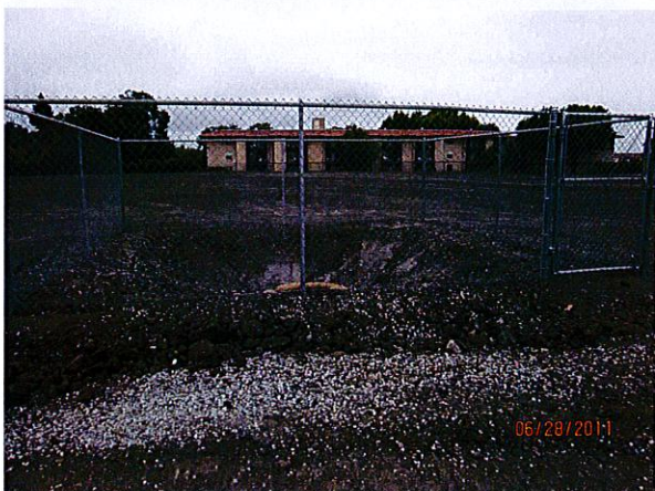
Fence installed around the protected well
