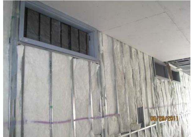
Framing, Insulation, Drywall & Window Frames
