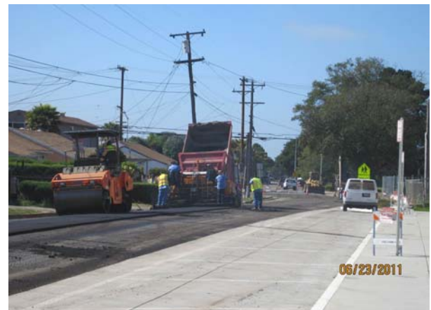
New AC Paving at 41st Street
