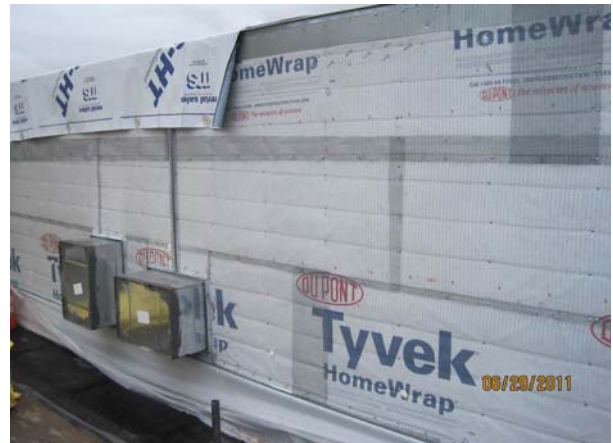
Tyvek & Chicken Wire at Roof Wall
