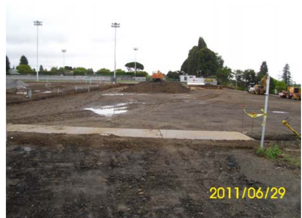
Existing access road removed and re-graded for tennis courts.
