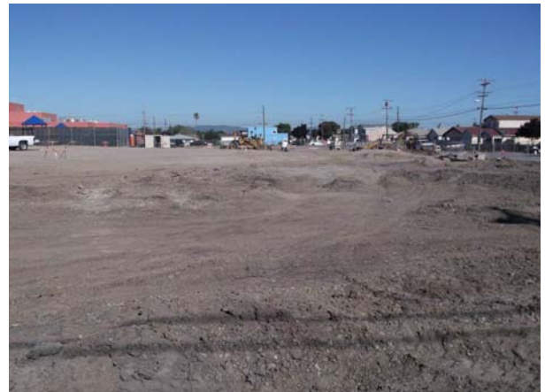
East Side of Site-Bldg. B & C Pad-COMPLETED
