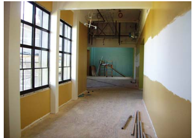
Interior Painting Nears Completion
