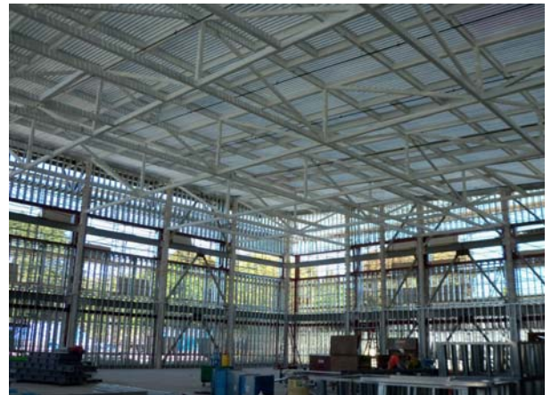
Building 8: Install Interior & Exterior Wall Framing
