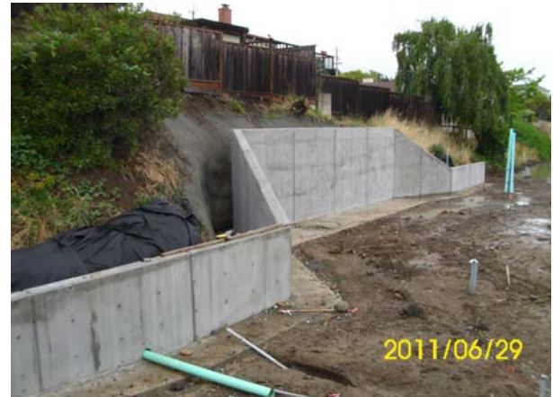
Main retaining wall complete behind baseball backstop
