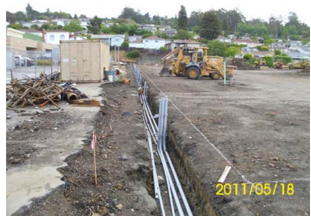
Underground electrical rough in for site lighting complete
