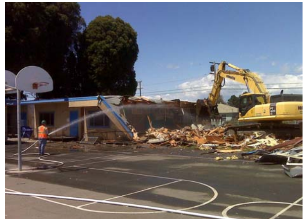
Demolition of Bldgs K1, K2, K3 & Portables-COMPLETED
