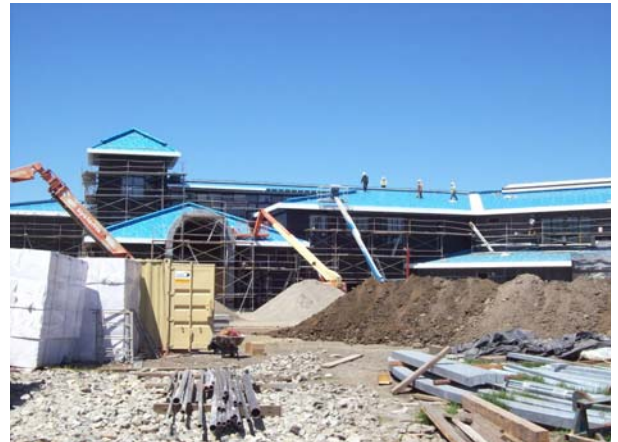
Roofing and Plaster Construction Advances
