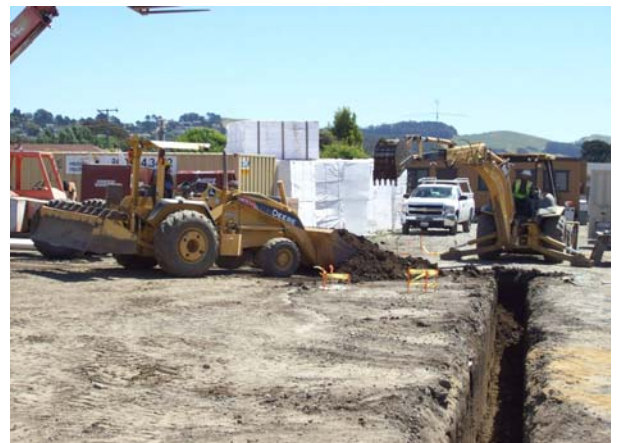
Underground Utilities Construction; Storm Drainage System
