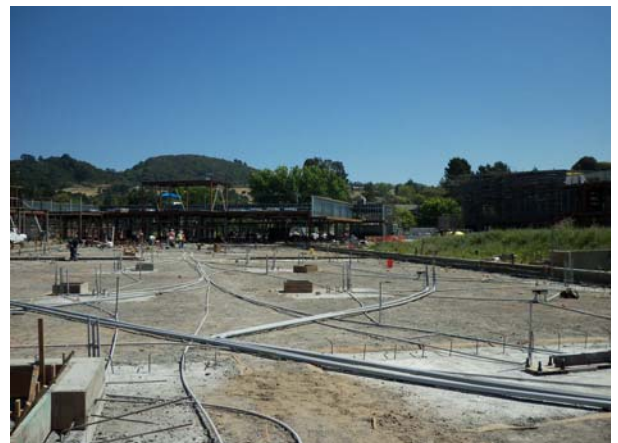
Building 7: Under-Slab Utilities Installation
