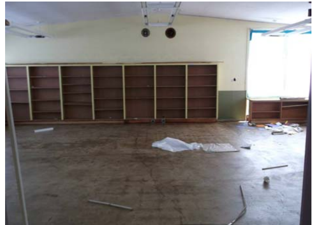
Abatement of Bldgs K1, K2, K3 & Portables-COMPLETED
