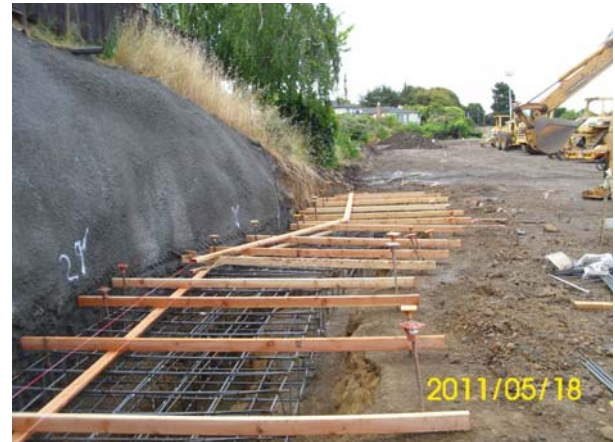
Shotcrete stabilization, rebar and footing for retaining wall
