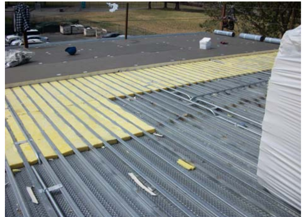
Installation of Batt / Base Sheet on flat roof
