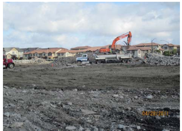
Off hauling of Concrete
