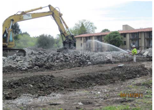
Processing the concrete
