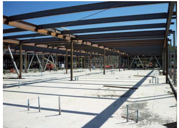
Building 6: Structural Steel Installation
