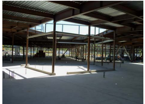
Building 4: Metal Roof Deck Installation
