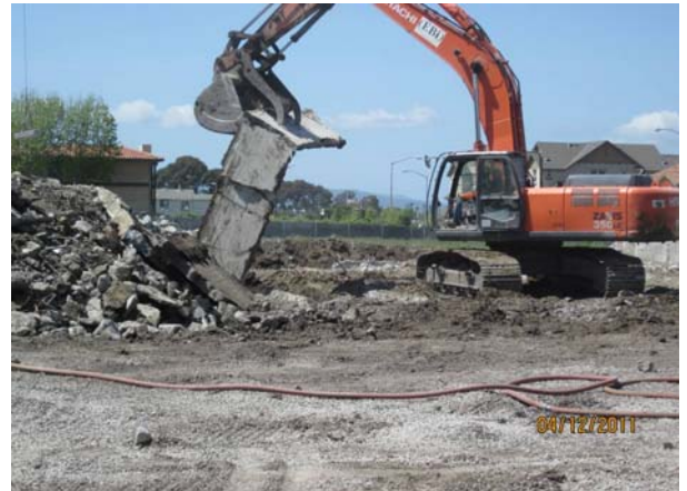
C-Bldg. - Demolition of slab and footings
