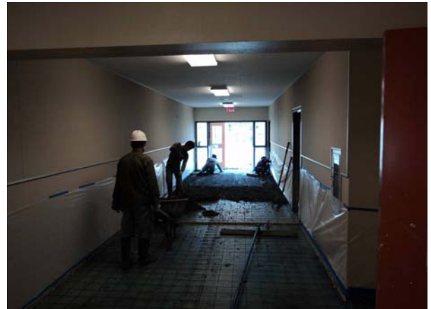
Light weight concrete installation
