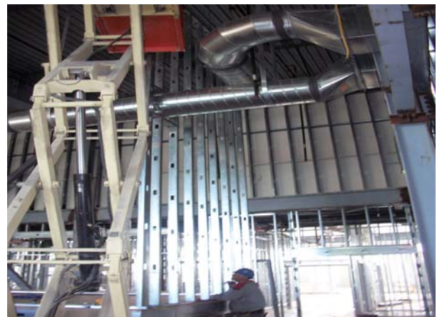
Full height framing at stage
