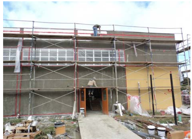
Stucco finish coat installation
