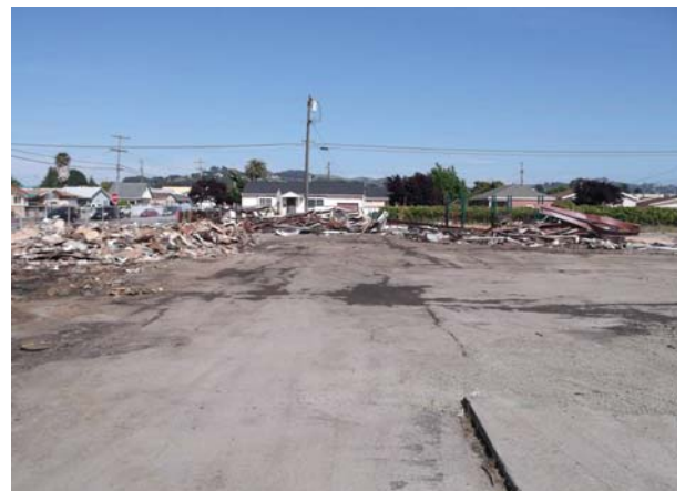
Removal of Site Debris-In Progress
