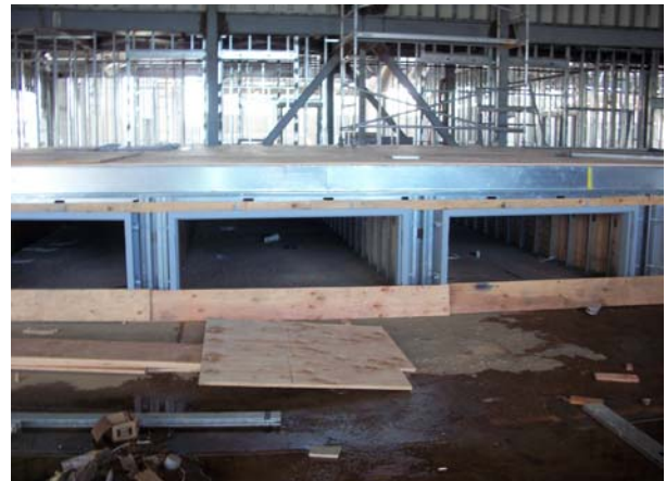
Stage Framing with Plywood
