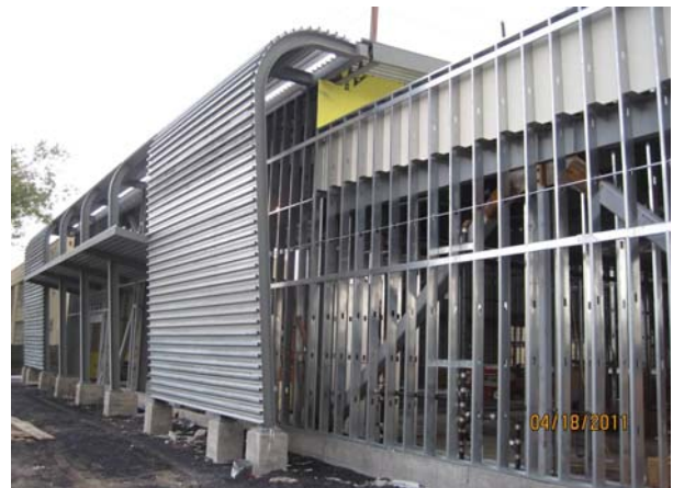
Exterior framing and metal panels
