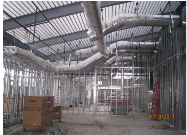
Stud framing, ductwork, sprinkler lines
