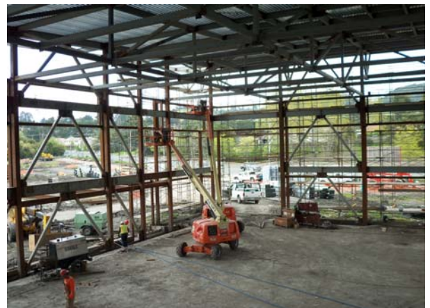
Building 8 Metal Roof Deck Installation
