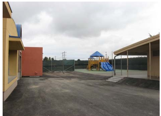
Bldg "A" Installation of Fence for Temporary Play Area
