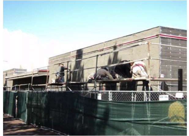
Stucco installation on building A-1
