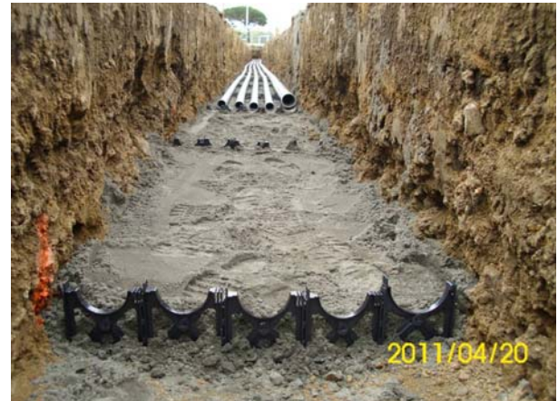
Utility Trench-Chair supports for electrical conduits
