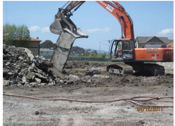
C-Bldg. - Demolition of slab and footings
