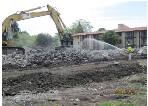
Processing the concrete
