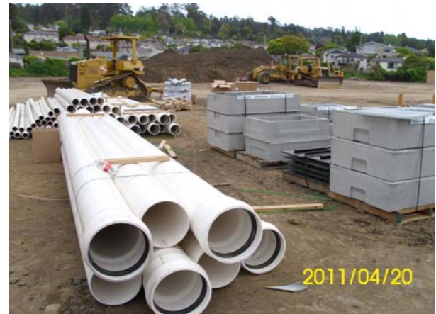
Drainage system materials on site
