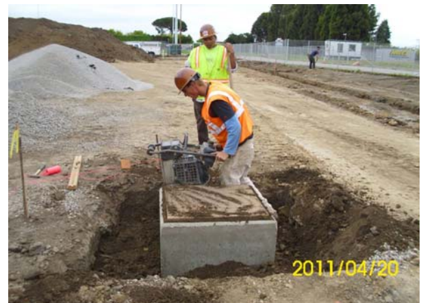
Installation of concrete drain inlet
