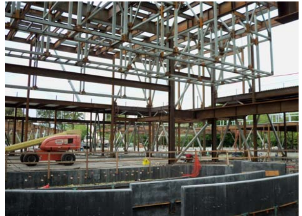
Building 2 Structural Steel Installation
