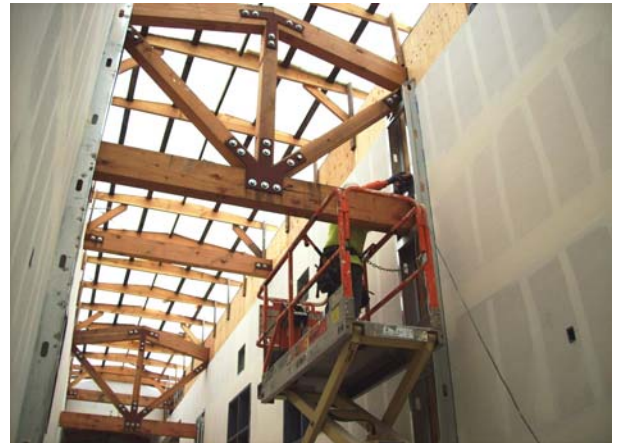
Area B; 2nd Floor Corridor @ Construction Continues
