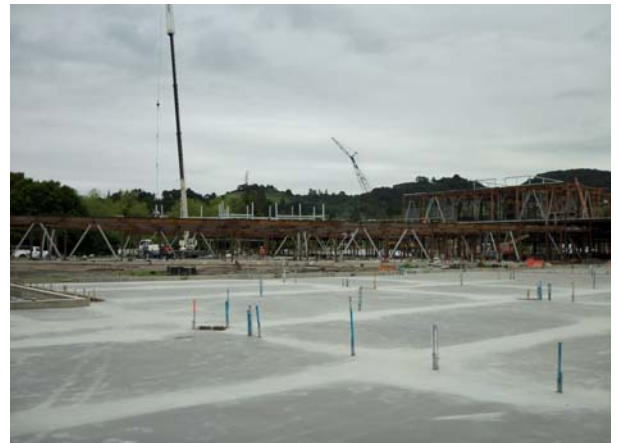
Building 6 Slab on Grade
