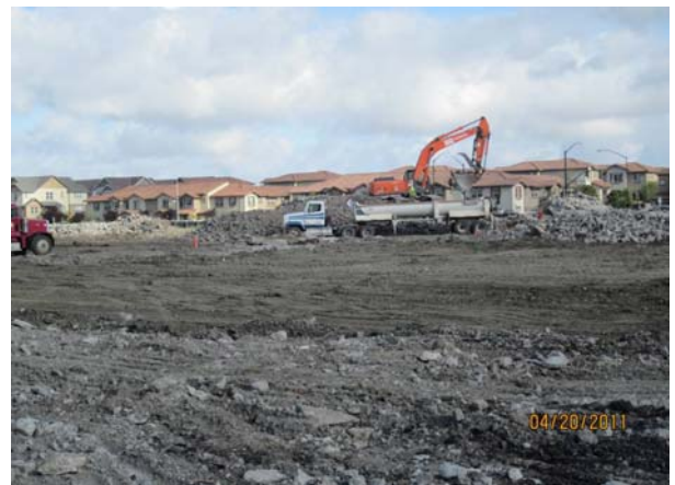
Off hauling of Concrete
