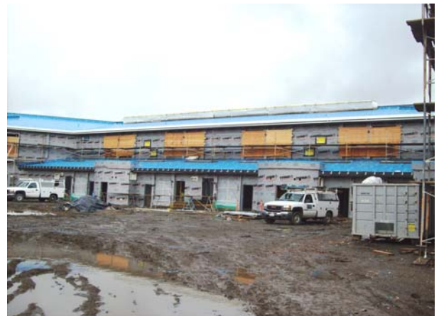
Area B; Final Building Wrap complete
