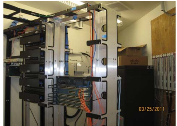
Electrical Equipments in MDF
