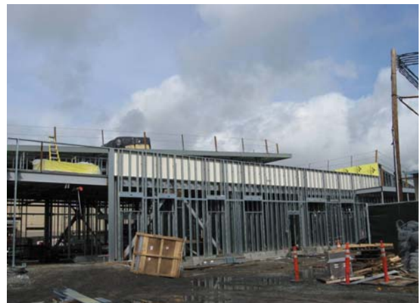
Exterior Framing and start of exterior DensGlass
