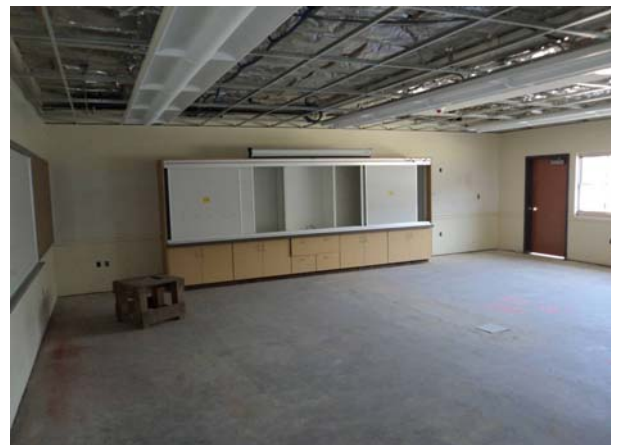
Casework installed in classroom
