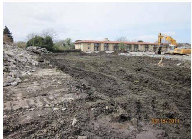
C-Bldg. - Demolition of slab and footings
