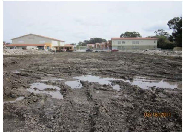
Gymnasium - Demolition of slab & footings
