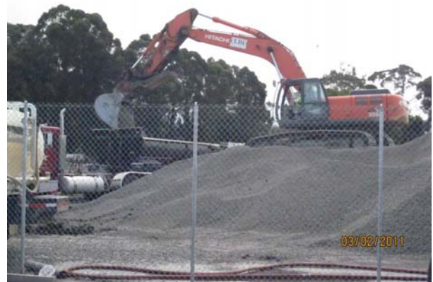
Off haul of processed concrete
