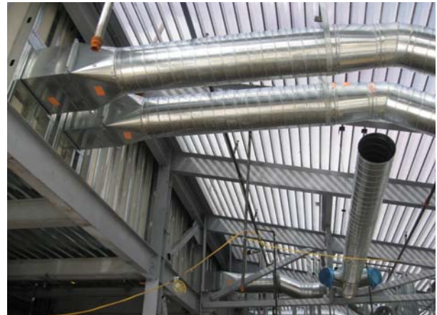
Installation of Ductwork
