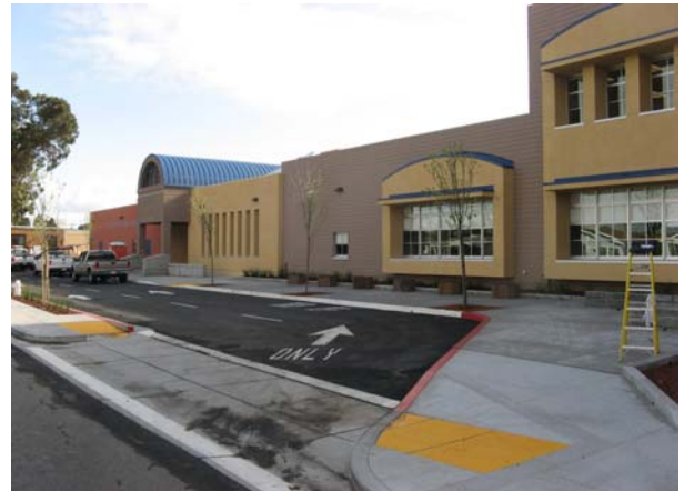
Bldg "A" Site Landscaping
