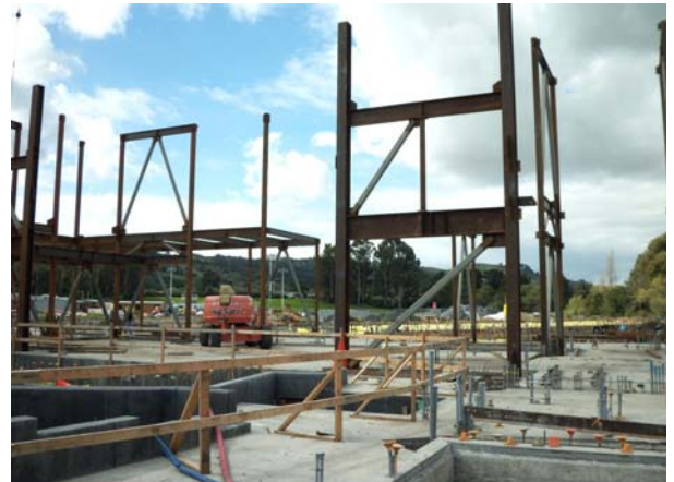
Building 2 Structural Steel Installation
