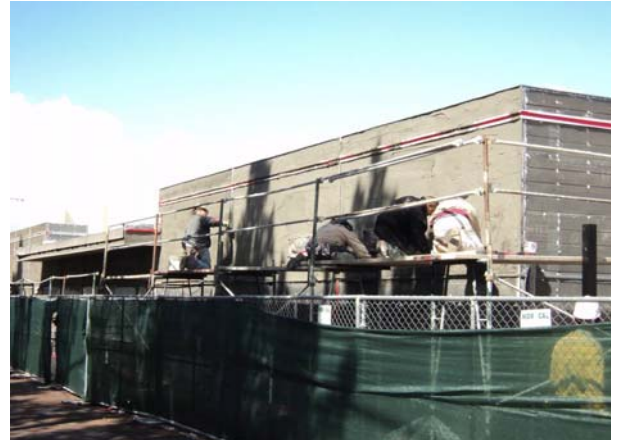
Stucco installation on building A-1
