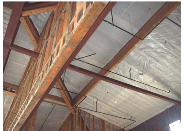
Area C, Multi-Purpose Room; Ceiling Insulation Near Complete
