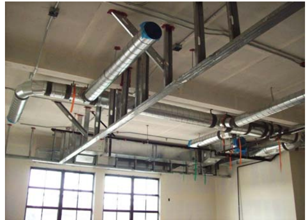
Area A; Ceiling Utilities, Soffits & Ceiling Frame Advance
