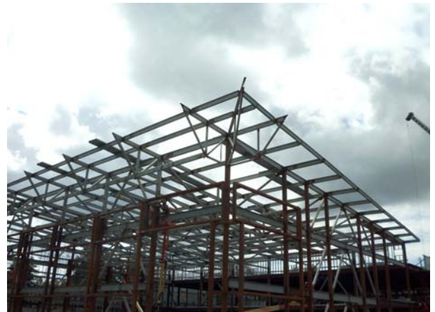
Building 8 Roof Truss Installation
