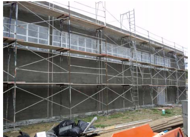
Stucco installation on Multi Purpose Room
