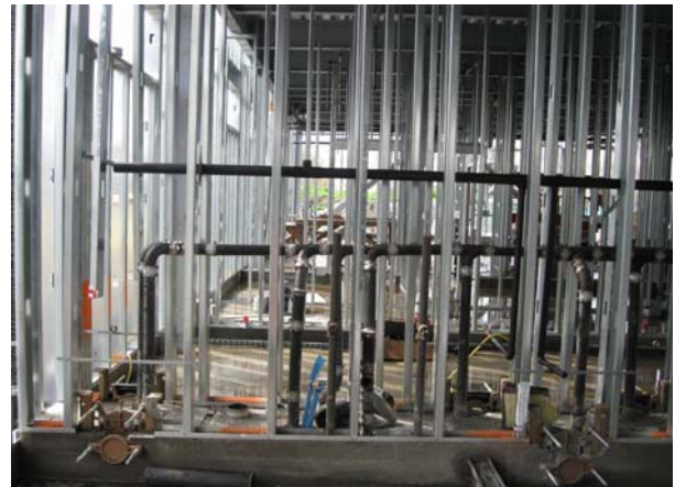
Installation of Restroom Plumbing / Interior Framing
