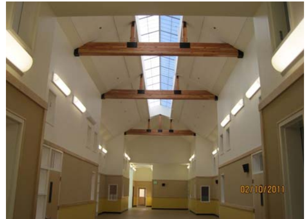
Building B - Corridor at 2nd Floor
