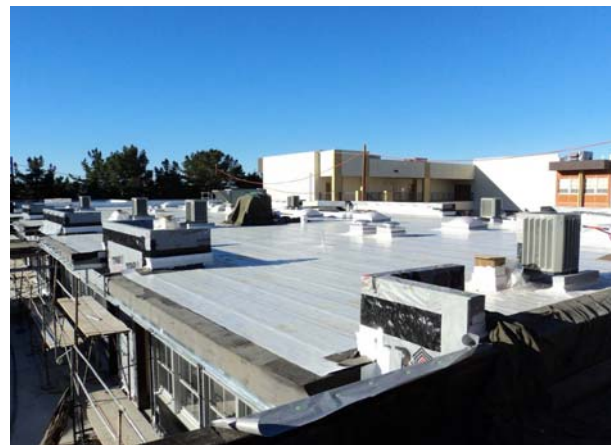
HVAC installed on building A-4
