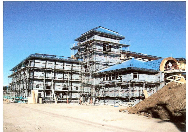
Area A: Exterior Waterproofing & Plaster Prep Advances
