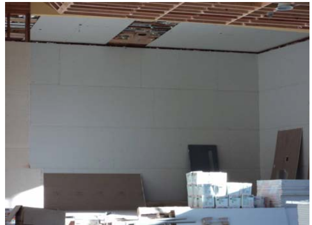
Drywall installation in Multi-purpose room and soffit.
