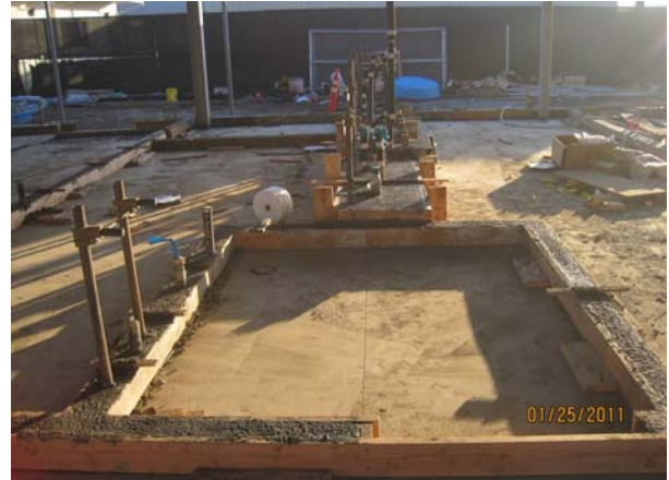
Curbs and Block-outs w/ Toilet Carriers
