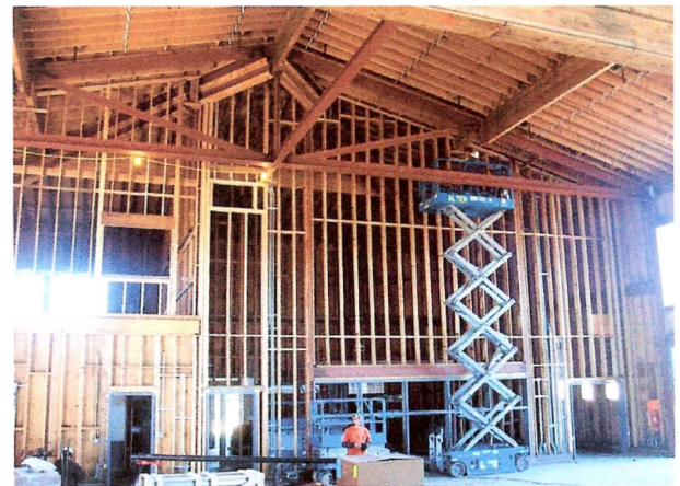
Area C, Multi-Purpose Room: Sprinkler System Underway
