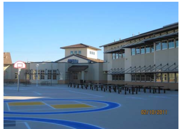
Site - Colored Asphalt Concrete & Striping
