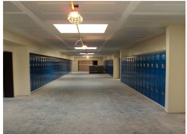
Lockers installed in building A-1
