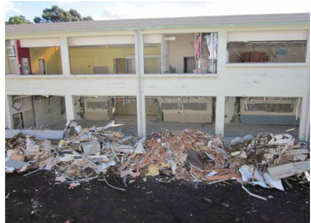
C Bldg - Interior Demolition
