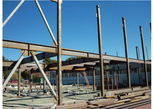
Building 8 Erect Structural Steel
