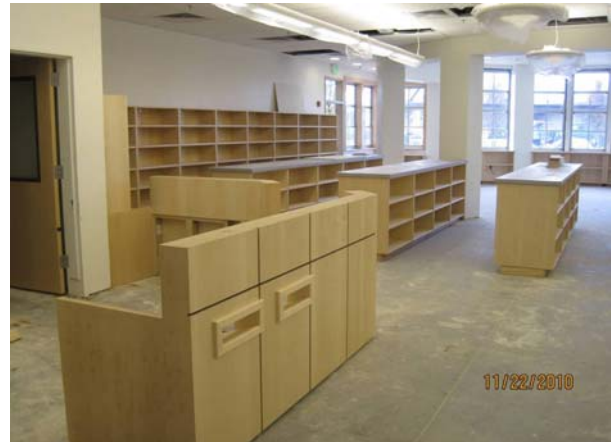
Building A: Library Casework
