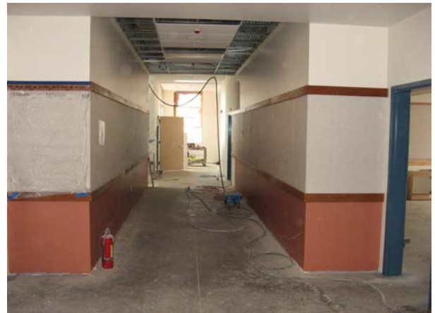
Bldg "A" (North) Corridor with Paint, Panels, and Trim
