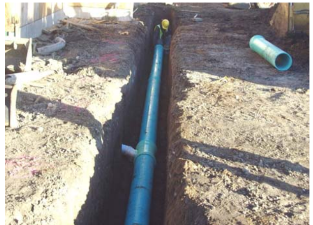
Underground Utility Construction Continues
