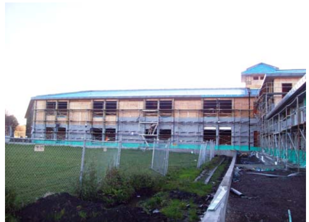
Exterior Wall and Window Development is Underway
