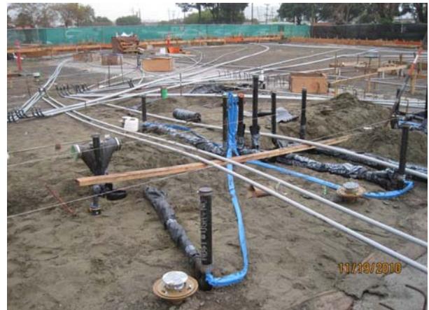
Under Slab Plumbing & Electrical
