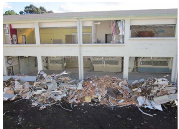
C Bldg - Interior Demolition
