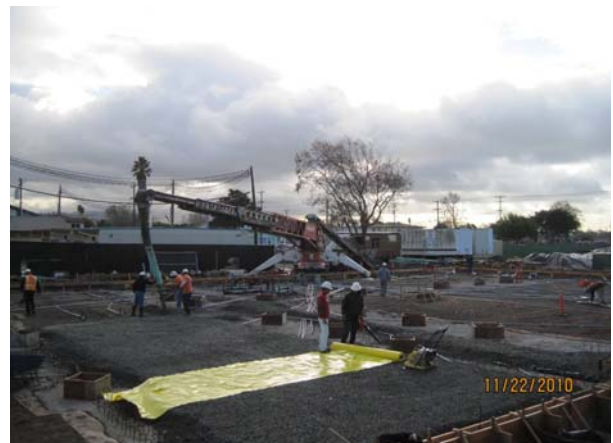
Gravel & Vapor Barrier Placement
