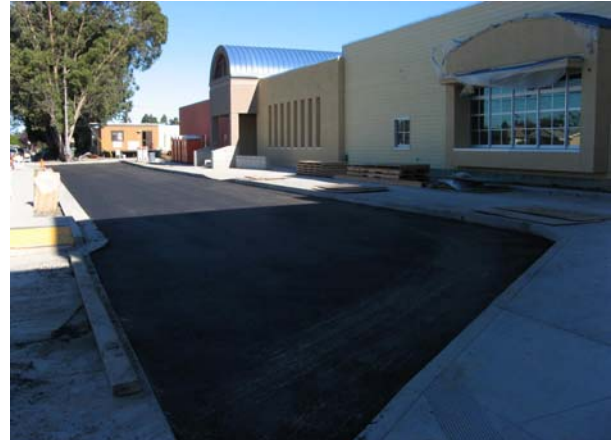
Bldg "A" New Curb, Sidewalk, Ramps, and Drop Off
