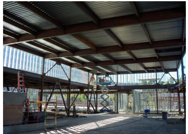
Building 9 Layout & Cut MEP Roof Penetrations
