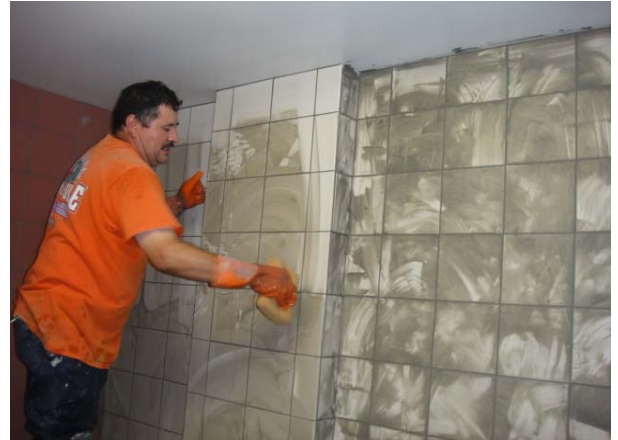
Grout work in coaches bathroom
