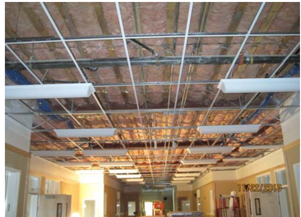
Building B: Light Fixtures & Sprinkler Drops
