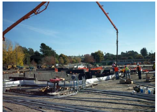
Building 2 Pour Concrete Slab for Seating Pit
