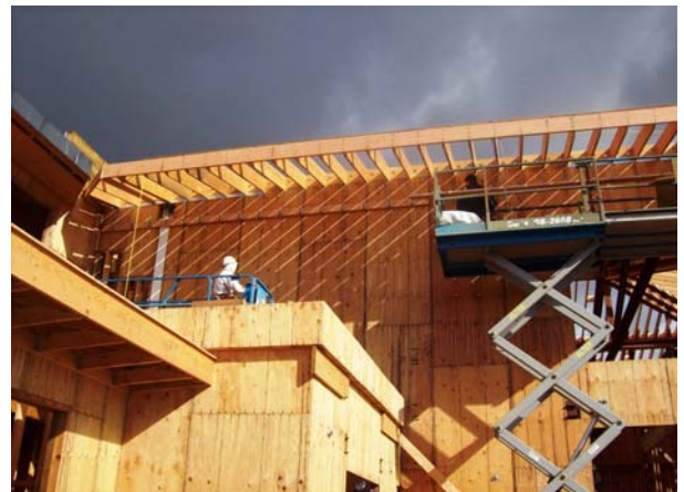
Area C - Construction of the Roof Soffet
