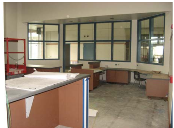
Bldg "A" (North) Installation of Interior Millwork
