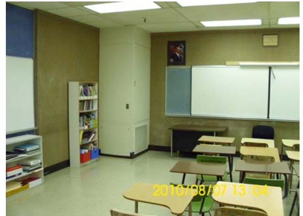
New Heating units in each classroom
