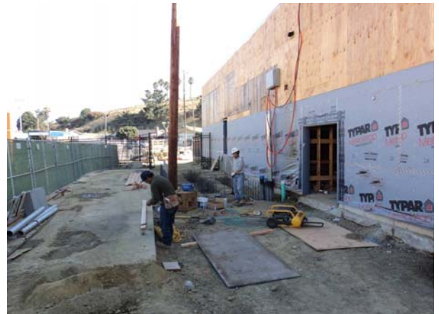
Footing for concrete ramp at Band Room
