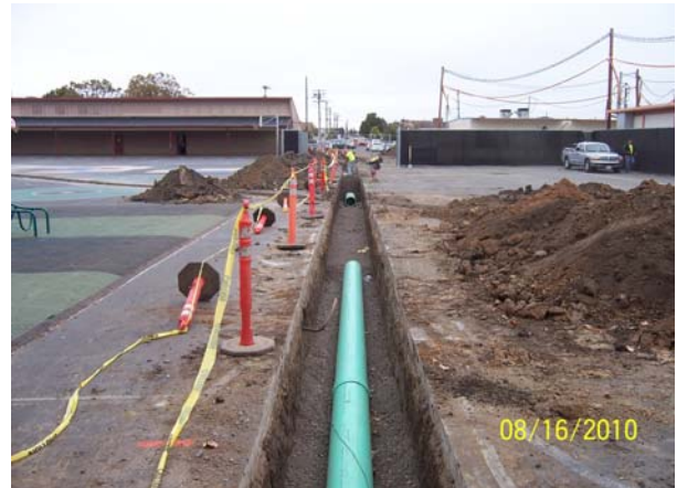
Storm Drain Line Install
