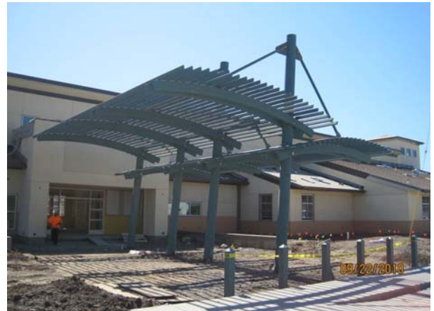
Building A Main Entrance: Canopy
