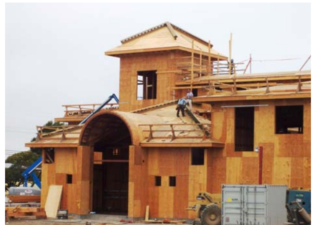
Area A - Library & Tower Roof Framing Near Completion
