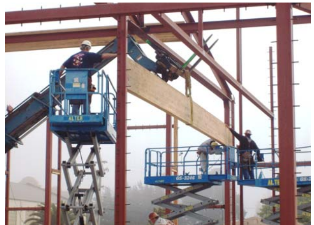
Area C; Glue-Laminated Beam Over Stage is Placed
