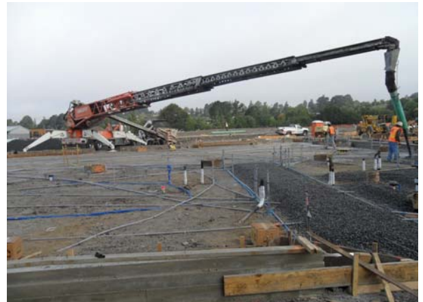
Building 9 Under-Slab Gravel Installation
