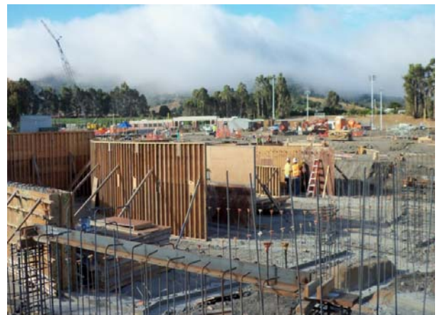
Building 2 Form and Rebar Walls
