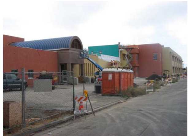
Bldg "A" Color Coat, Stucco, Siding, and Metal Roof
