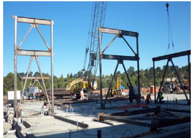
Building 9 Structural Steel Installation
