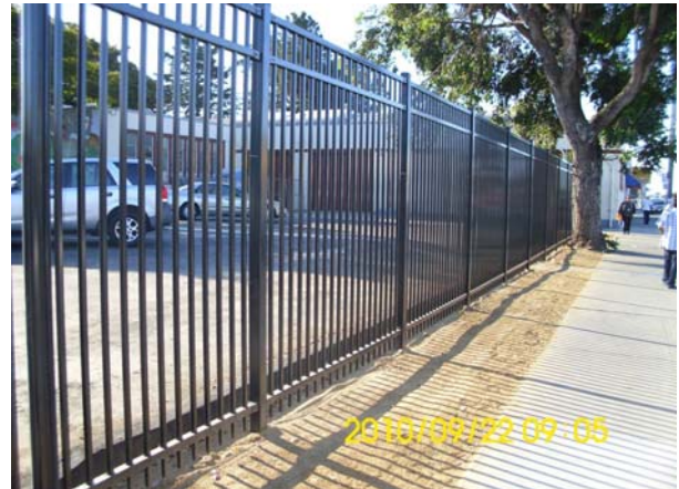
New ornamental fence at 23rd street
