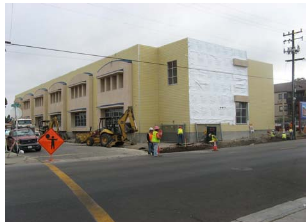
Bldg "A" (South) Install Siding and Sitework
