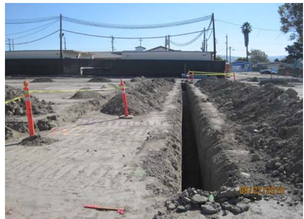
Underground Plumbing Excavation
