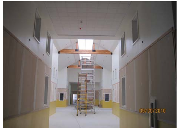
Building B 2nd Floor: Ceiling Tiles & Tack-wall
