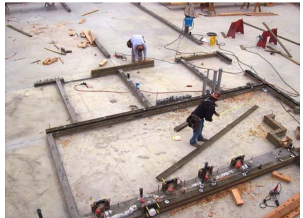
Area C - Wall Plate Placement @ Concrete Floor Curbing
