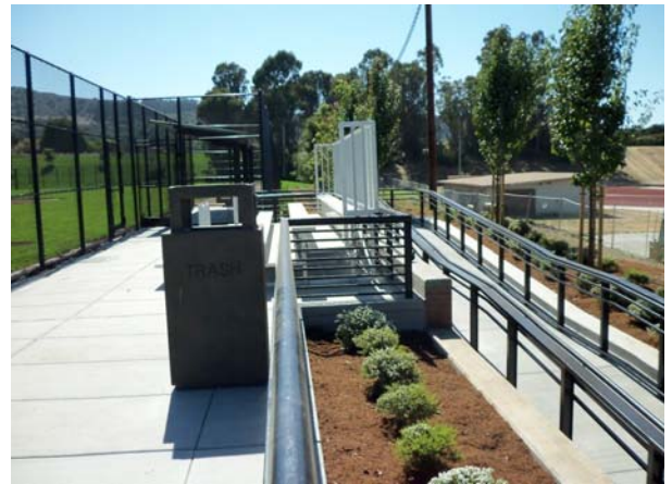
Installation of Guard Rails
