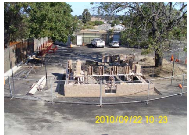
New Trash Enclosure under construction
