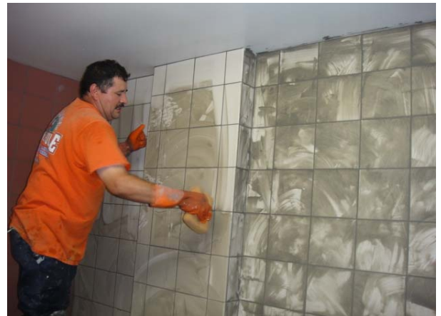
Grout work in coaches bathroom
