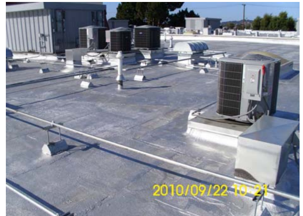
New Condensing Units (Air Conditioning) to each classroom
