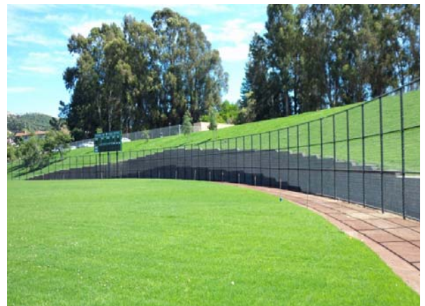
Anti-Graffiti Installation on Keystone Wall
