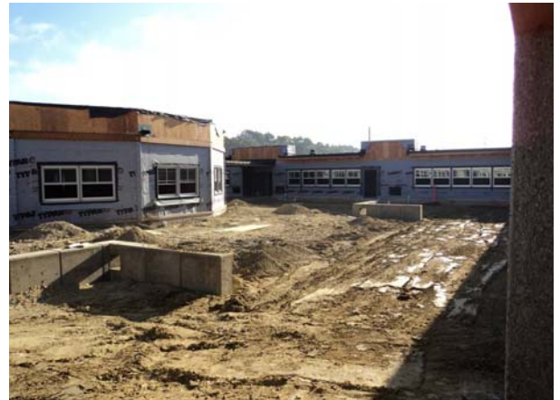
sub grade prep for courtyard
