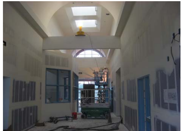
Bldg "A" (North) Install-Gyp Board, Mud &Tape, Int. Paint
