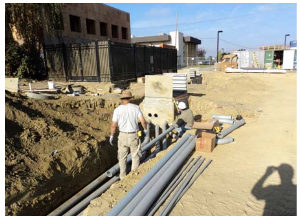
Power and data systems conduit installation
