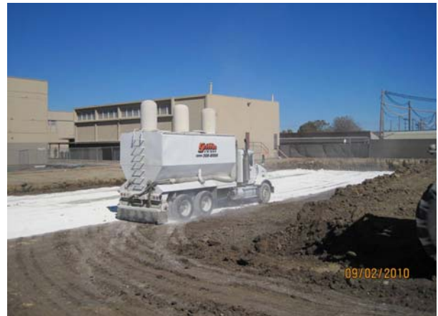
Building Pad Lime Treatment
