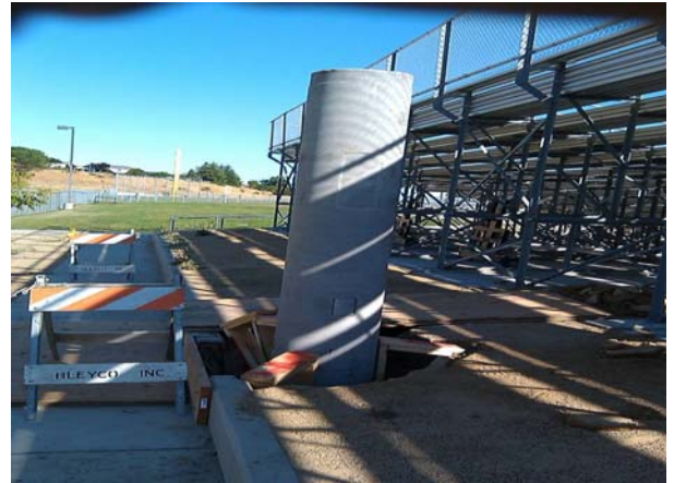
Installed Foundation Base at F-4
