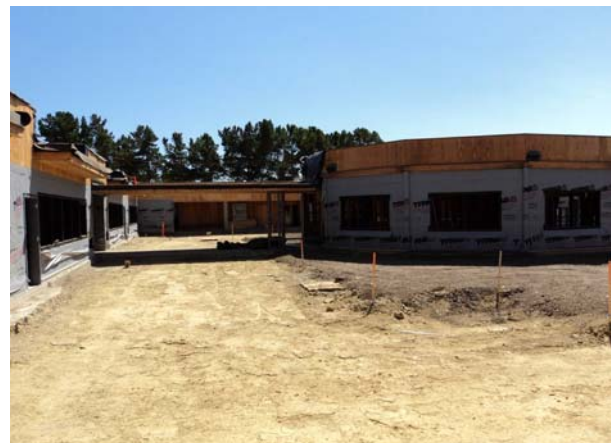
Finish graded courtyard ready for utility installation
