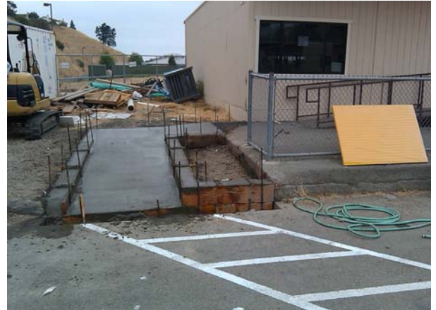
ADA Ramp at South End of Portables looking west
