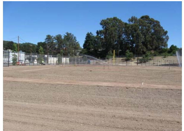
Playing Field Sod Installation & Irrigation System Testing
