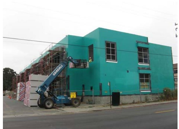
Bldg "A" (South) Lath & Plaster/Window/Bldg Waterproofing
