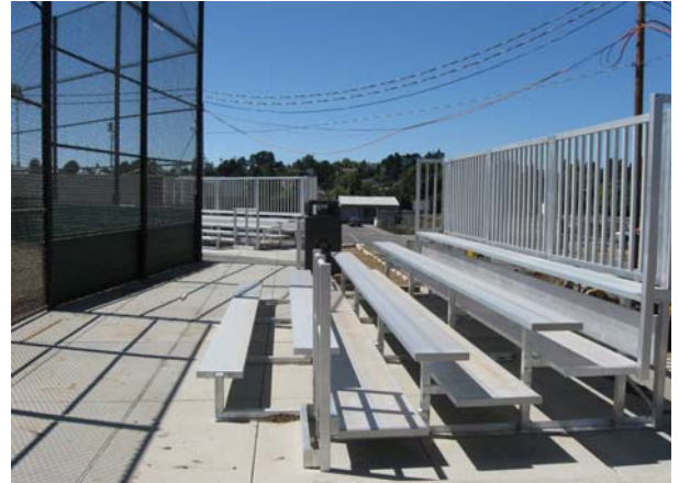
New Bleacher Installation
