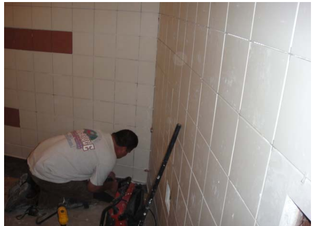
Ceramic Tile - Bldg. A Bathroom
