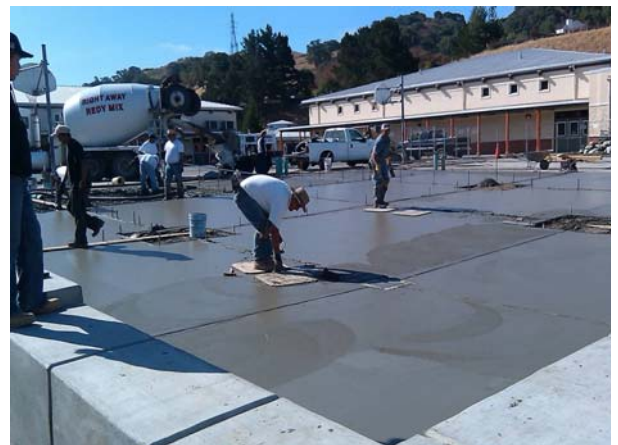
Placing of Concrete at Patio Area
