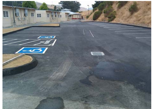
Completed Teacher's Parking Lot
