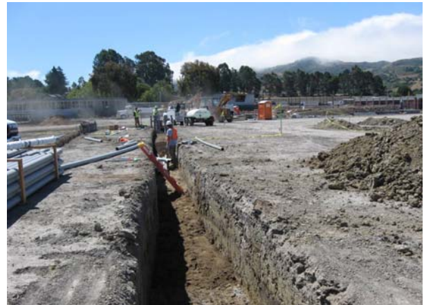
Site Electrical Utilities Installation
