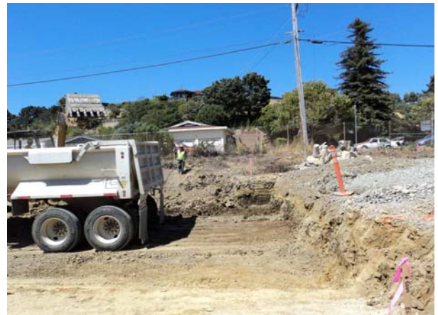
Expansive material removal in parking lot
