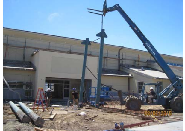
Building A Main Entrance: Canopy Steel
