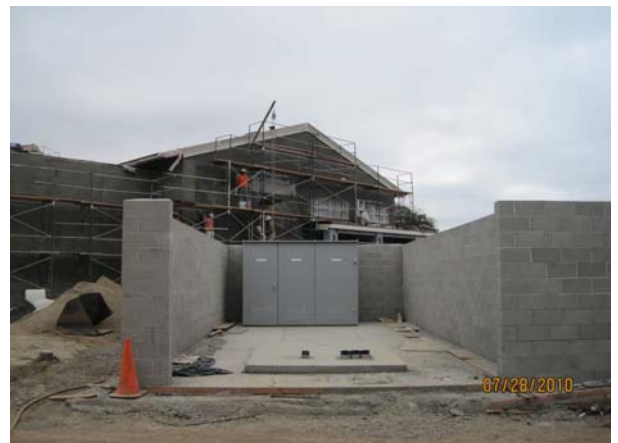
Site: Transformer Pad w/ Stucco Work at C
