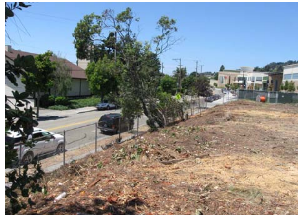
Trees Removed along Ashbury Ave.
