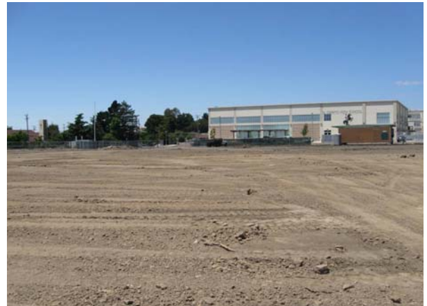
Excavation/Grading of Old Campus
