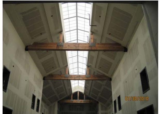
Building B 2nd Floor: Skylight
