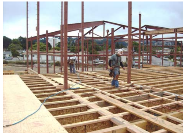
Area B; Blocking of 2nd Floor Joists Continues
