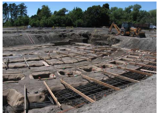
Building 2 Theater Footing Rebar Installation
