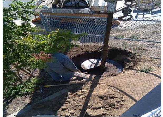
Drilling Pole Foundation at F-2
