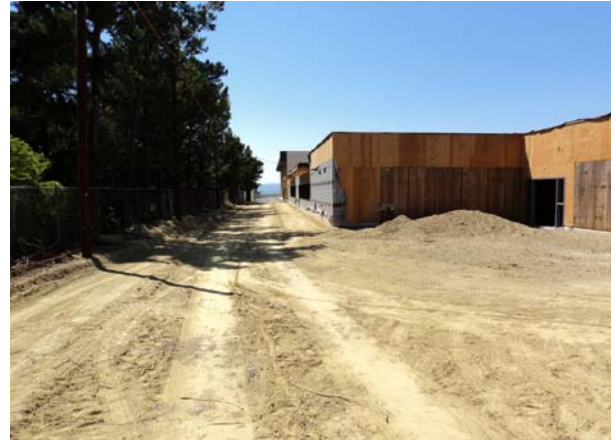
Rough graded fire access road
