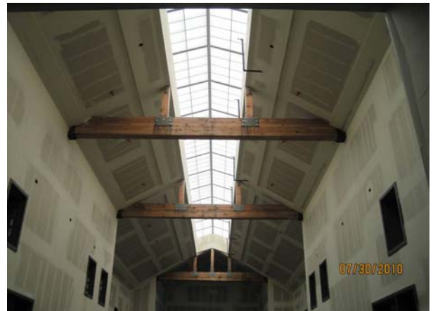
Building B 2nd Floor: Skylight
