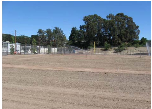
Playing Field Sod Installation & Irrigation System Testing
