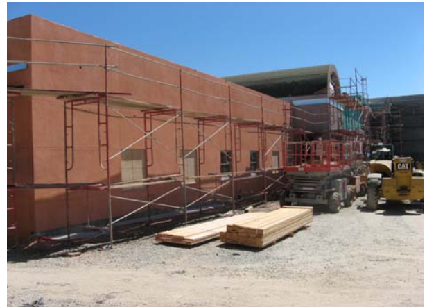
Bldg "A" (North) Color Coat on Exterior Stucco
