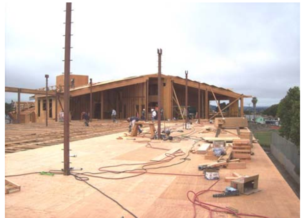
Area B; 2nd Floor Joists & Decking Progress
