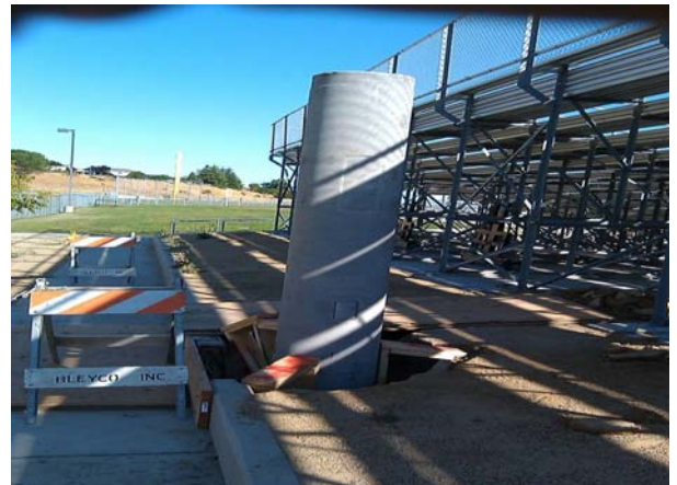
Installed Foundation Base at F-4
