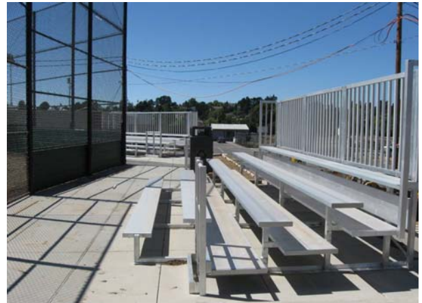
New Bleacher Installation
