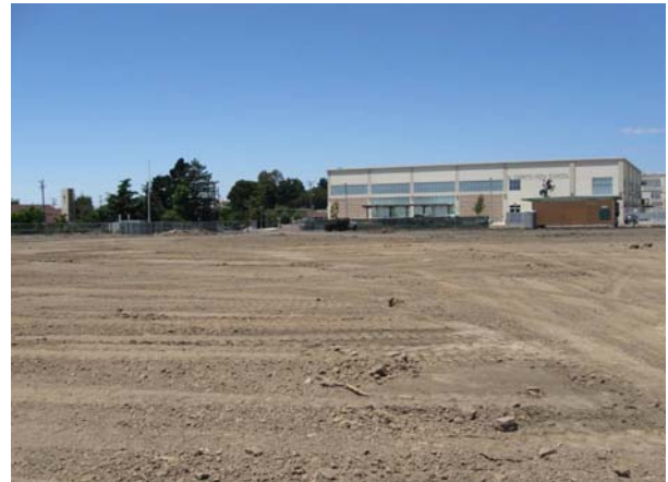
Excavation/Grading of Old Campus
