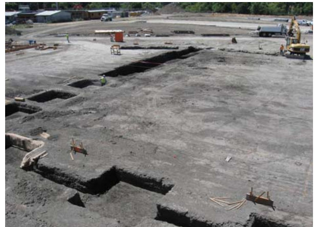
Building 8 Gymnasium Footing Excavation
