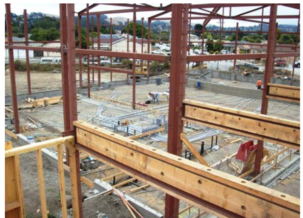
Area C; Underslab Electrical Utility Advances
