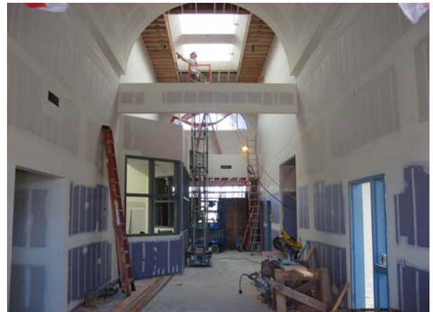
Bldg "A" (North) Install-Gyp Board with Mud and Type
