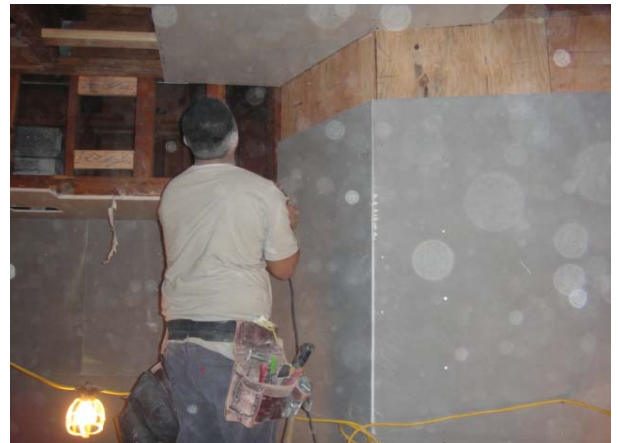
Drywall - A Bathroom
