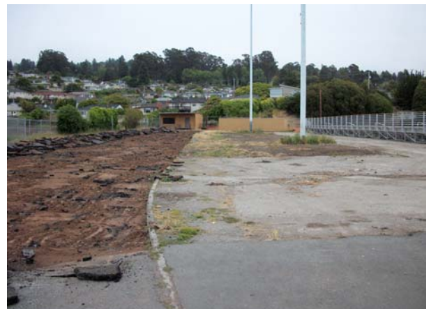
Containers Removed from Field
