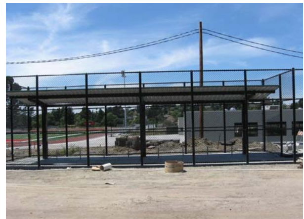
Installation of New Shade Structure
