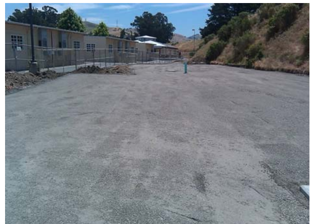
Final Grading of Teacher's Parking Lot
