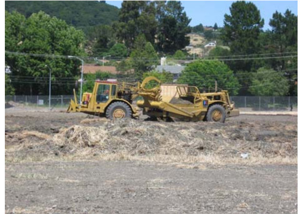
Site Clearing & Grub Removal
