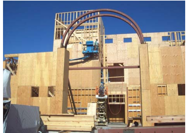
Area A (North); Exterior Wall Sheathing Progresses
