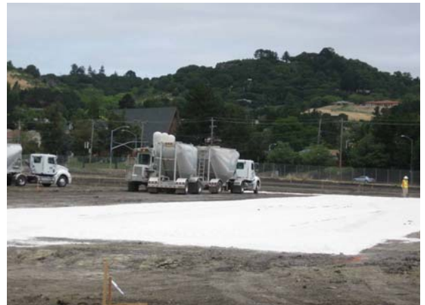
Lime Treatment of Building Pad
