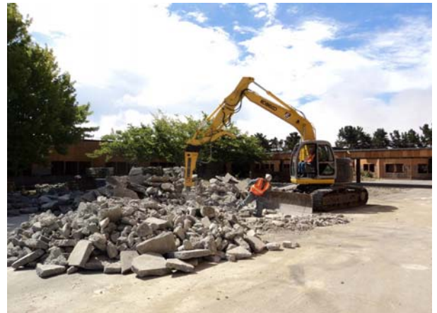
Main entrance demolition
