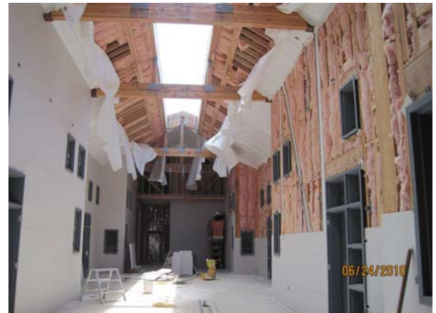
Building B 2nd Floor: Gypsum Board at Walls
