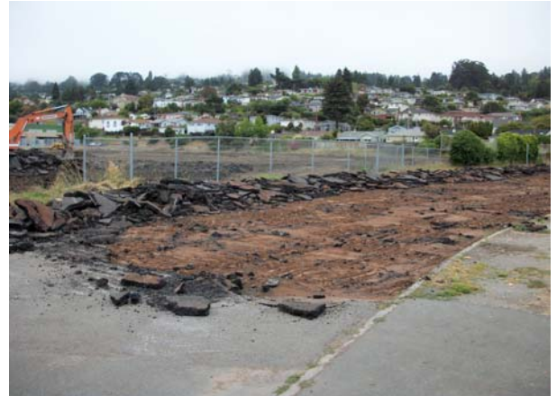
Asphalt Removal at Basketball Courts
