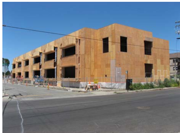
Bldg "A" (South) "Pop Outs" & Mech. Installation
