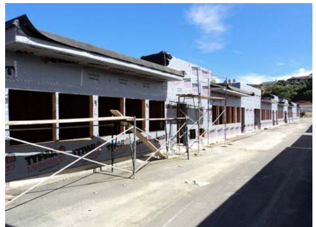
Stucco underlayment installation
