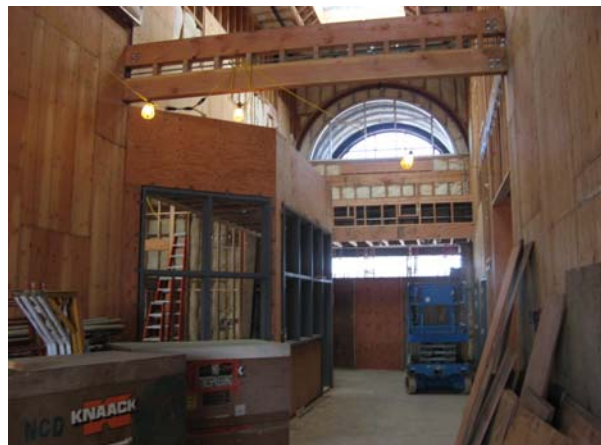
Bldg "A" (North) Install-Door/Window Frames & Insulation
