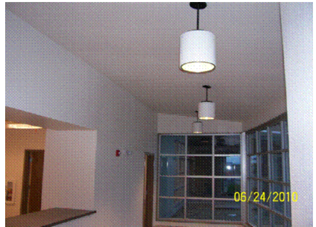
Main Lobby w/Storefront Windows & light Pendant Fixtures
