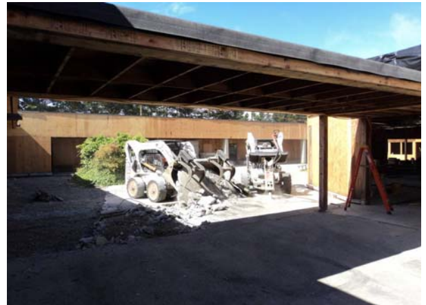
Court yard demolition
