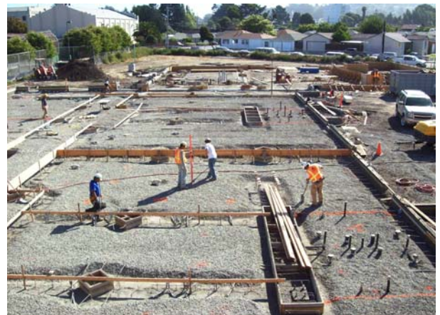
Areas B; Dressing of Base Rock for Slab-On-Grade Underway
