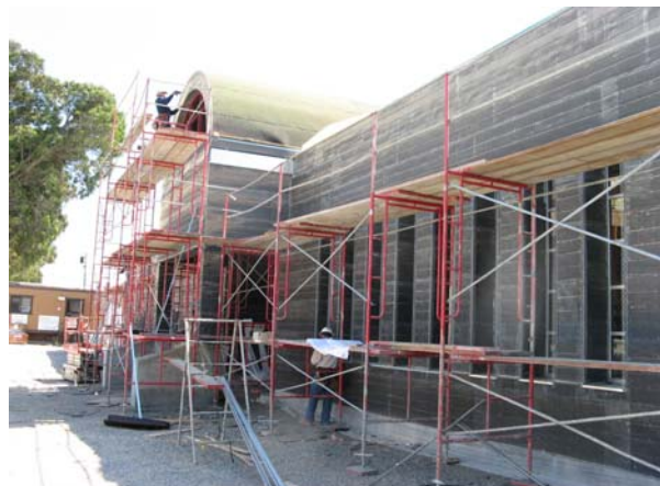
Bldg "A" (North) Installation of Lath for Plastering
