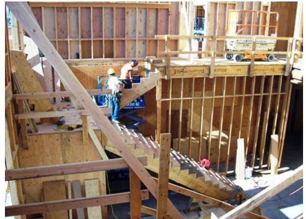
Area A (North); Stairway 2A & 2B @ Main Lobby Progresses
