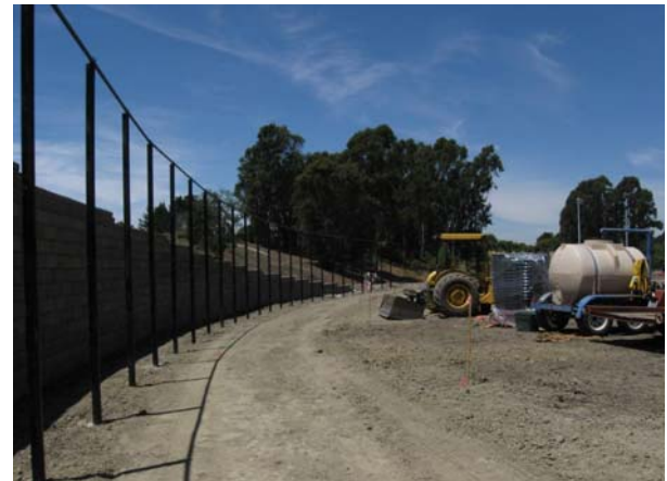
Installation of New Fencing and Backstop
