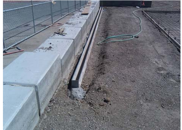
Foundation Walls & Drain at Quad Court Yard
