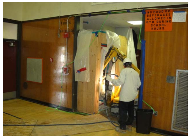
Mobile Jackhammer - Boy's Gym Bathroom
