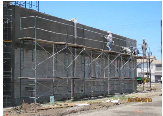
Building A East: Stucco - Brown Coat
