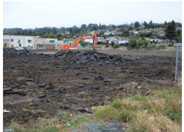
Temp Campus Asphalt Removal
