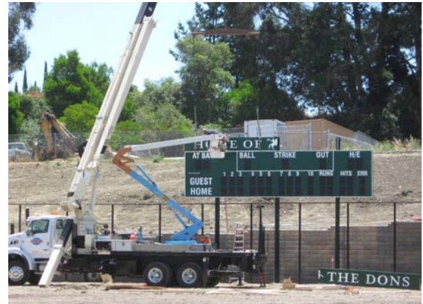
Installation of New Scoreboard
