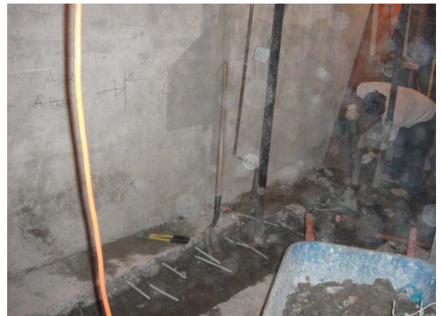
Slab Demo. Coach's Bathroom
