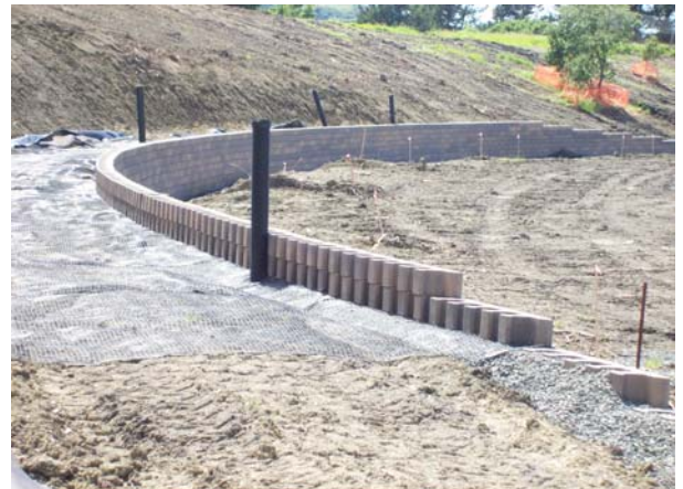
Modular Concrete Retaining Wall Excavation & Backfill
