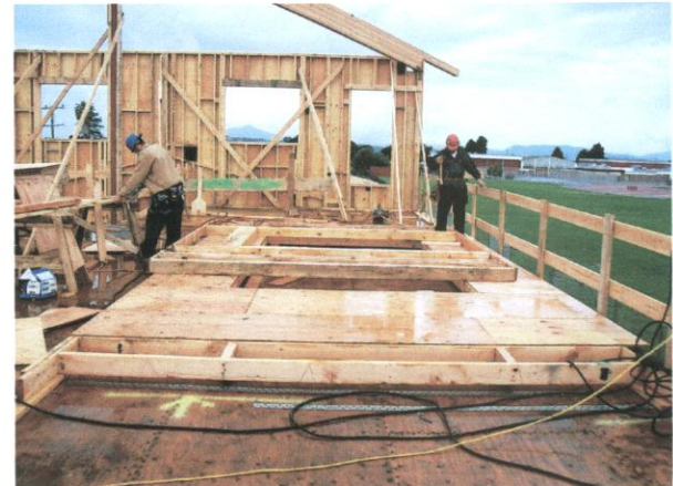
Area A (West); 2nd Floor Exterior Wall Fabrication
