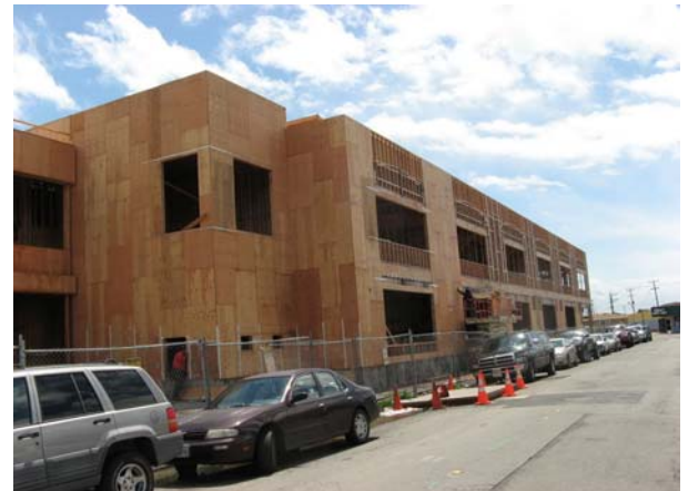
Bldg "A" (South) Installation of Ext. Plywood Sheathing
