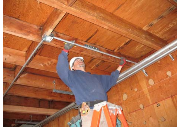
Installing electrical conduit in building A1
