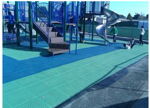
Highland A @ 100% Complete
