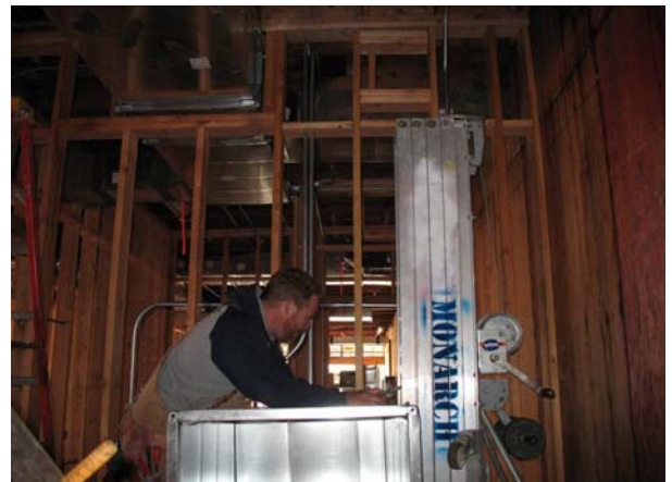
Mechanical installing in building A1
