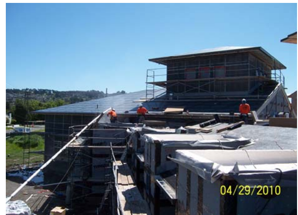
Building A East: Low Slope Roof Installation
