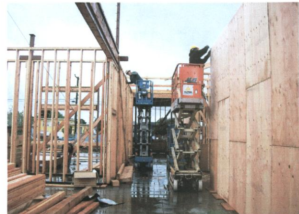
Areas B (East) - Framing along Corridor - View to South
