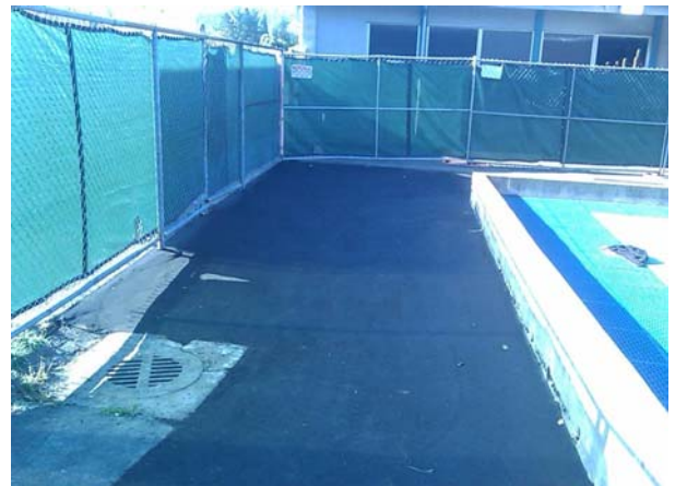
Valley View re-working of paved area
