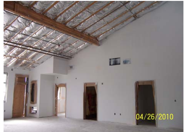
Building A West: Paint Primer
