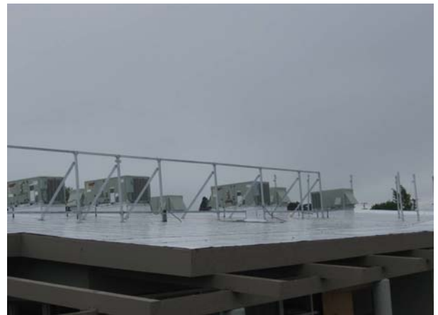
Mechanical Screen frames for HVAC Units
