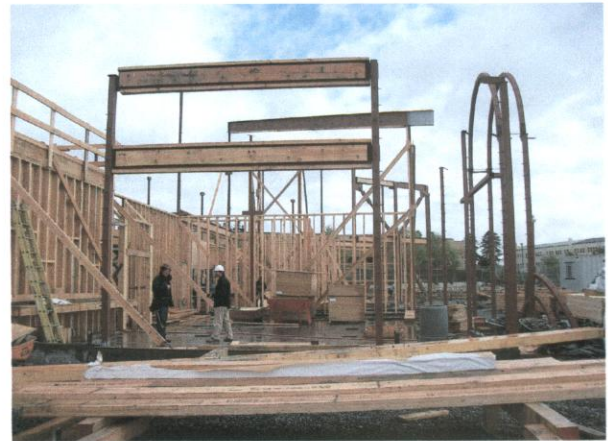
Area A (East); Framing Advances - View to Library
