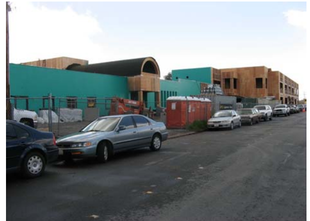
Bldg "A" (North) Application of Waterproof Membrane
