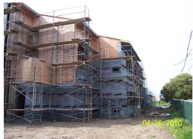
Building B: Metro wrap Building Paper
