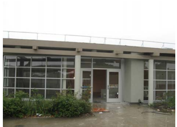
Storefront Windows & Doors at Main Entry
