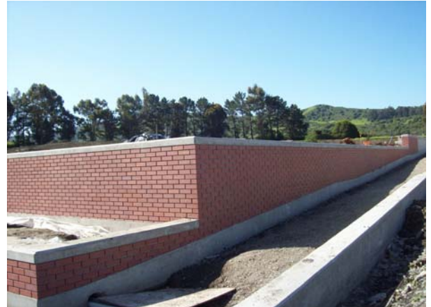
Installation of Brick Veneer at Concrete Retaining Wall
