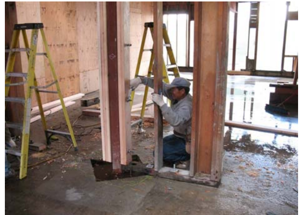
Rough framing at structural beam in building A3
