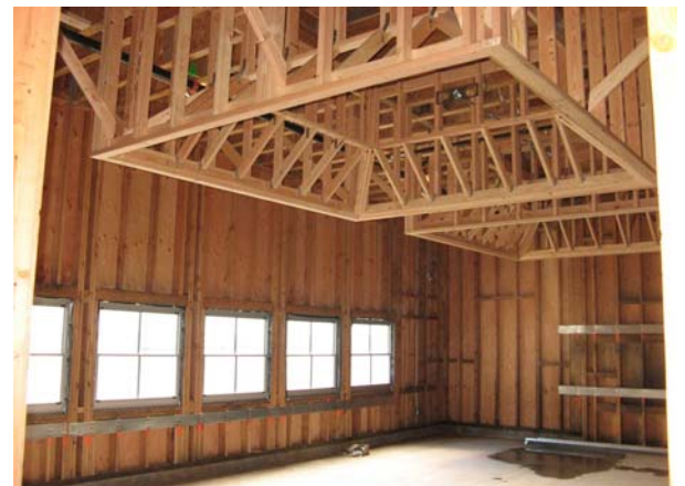
Bldg "A" (North) Installation Window Assembly & Skylite Frame
