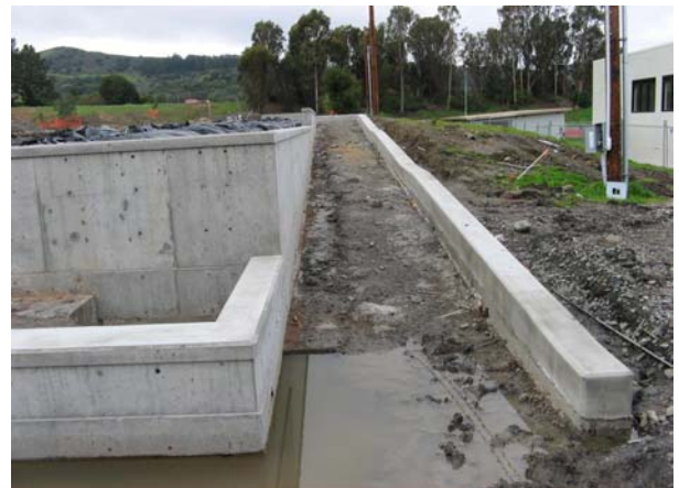
Construction of (N) Baseball Field Retaining Wall
