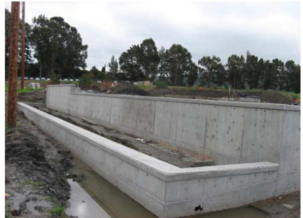
Construction of Baseball Field Retaining Wall
