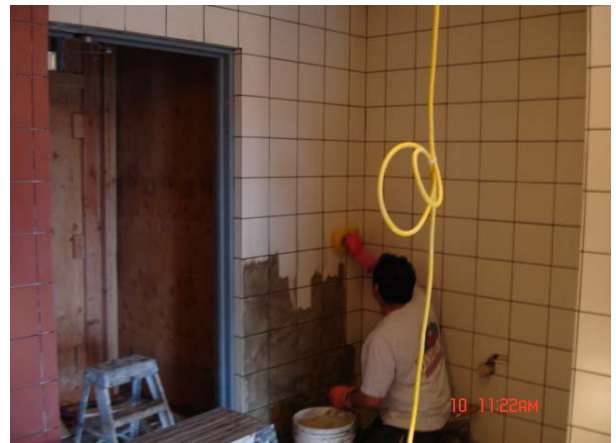
Wall Grout Work - Bathroom 700-6
