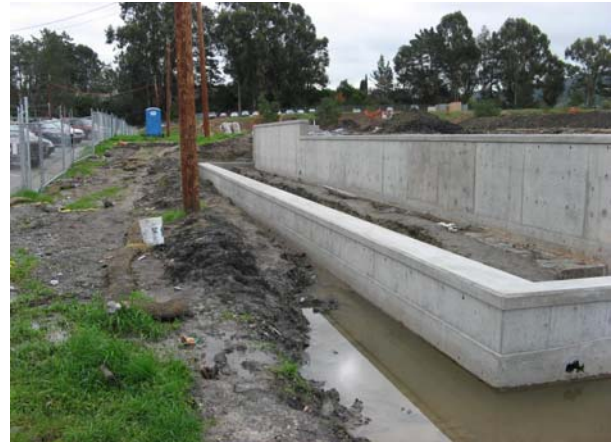
Construction of Baseball Field Retaining Wall
