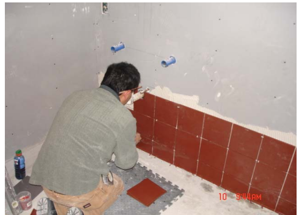
Wall Tile Installation - Bathroom 800-3
