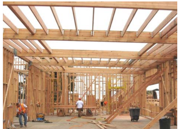
Installation of 2nd Floor South Roof Framing System
