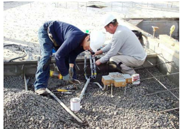
Areas B (East) - Underslab Utilities Nears Completion
