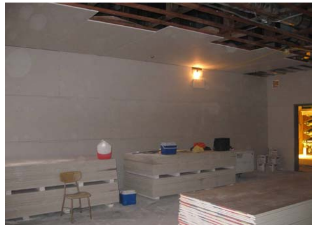
Sheetrock Walls/Partial Ceiling
