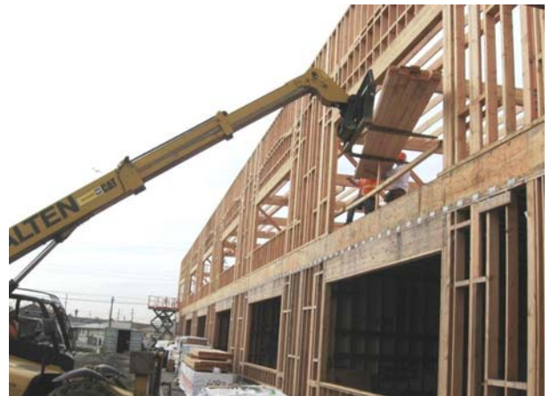
2nd Floor South Exterior Wall Framing
