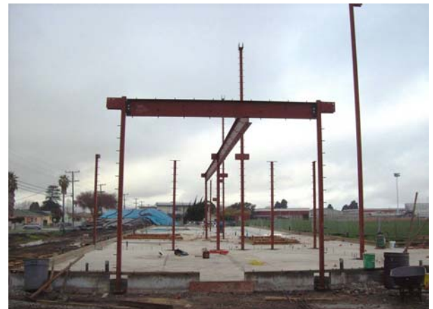
Area A (West) - Construction Advances to Framing
