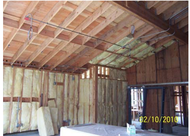
Building A: Gypsum Board Delivery & Batt Insulation Install
