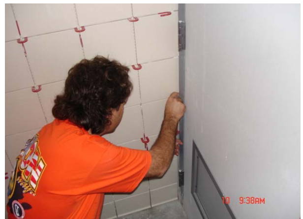
Wall Tile Alignment - Bathroom 800-2
