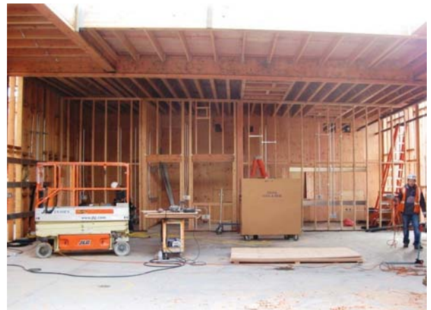
Installation of North Interior Wall Sheathing
