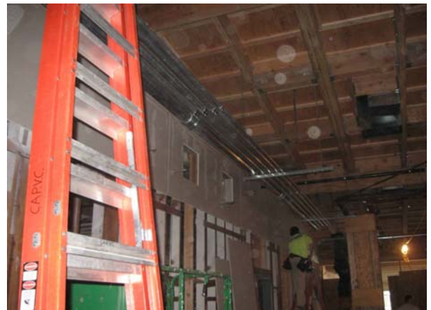
Run Conduit/Duct Drops/Sheetrock 1-Side
