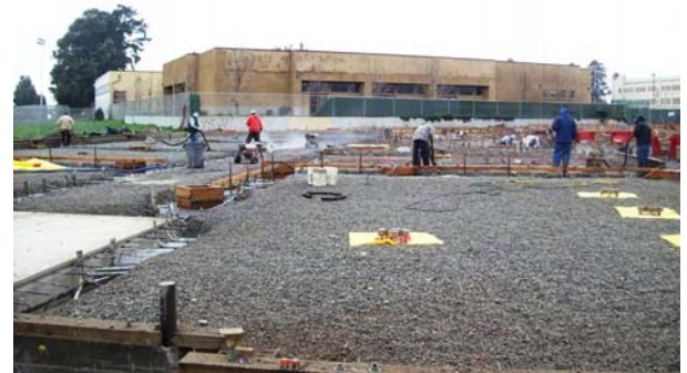
Area A (East) - Slab-On-Grade Preparation Advances
