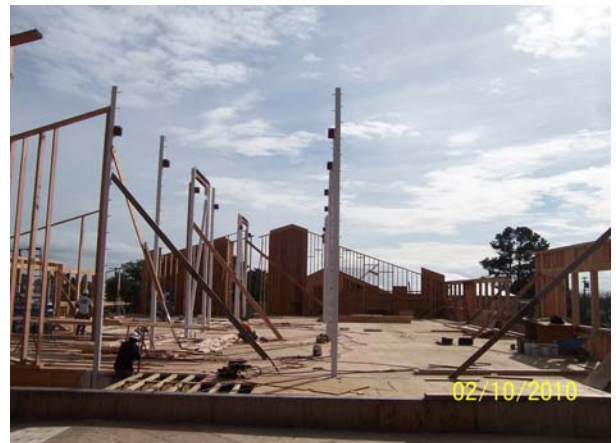
Building B: Second Floor Framing
