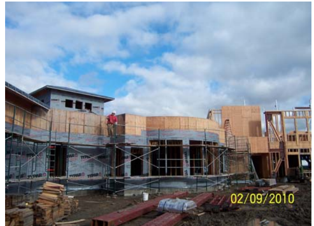
Building A: Exterior Scaffold & Building Envelope
