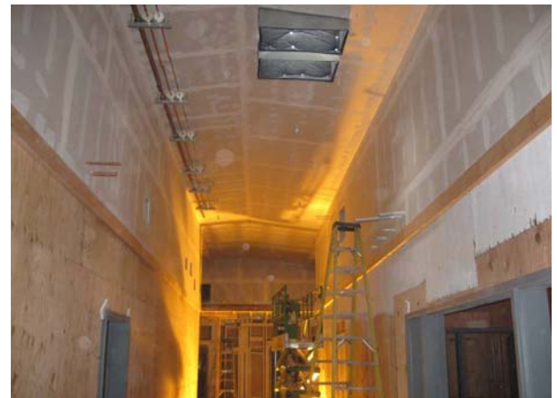
Sheetrock Ceiling/Duct Drops
