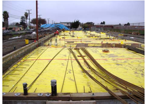
Area A 1st Slab-On-Grade Preparation Advances
