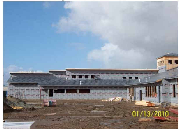
Building A: Waterproof Underlayment & Building Envelope
