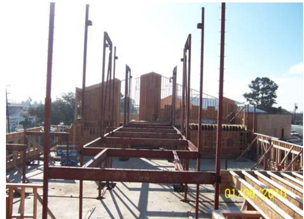
Building A: Flat Roof with Mechanical Curbs & Skylight
