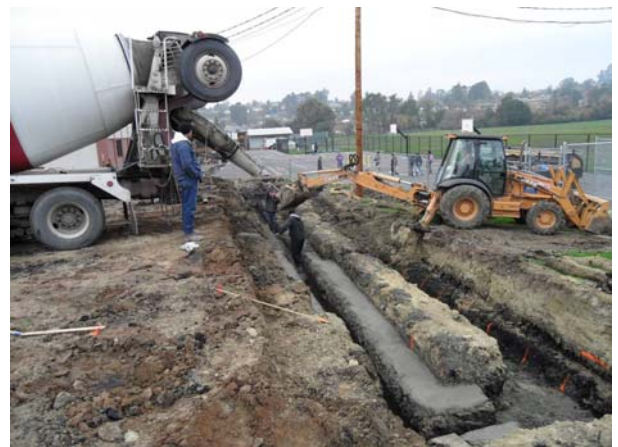
Construction of Baseball Field Retaining Wall Foundation
