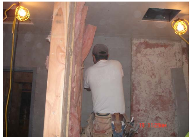
Hanging Drywall - Bathroom 800-2
