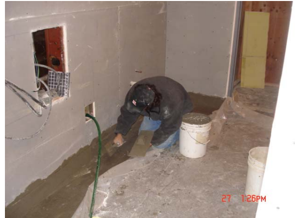
Mortar Bed at Wall Base - Bathroom 700-2
