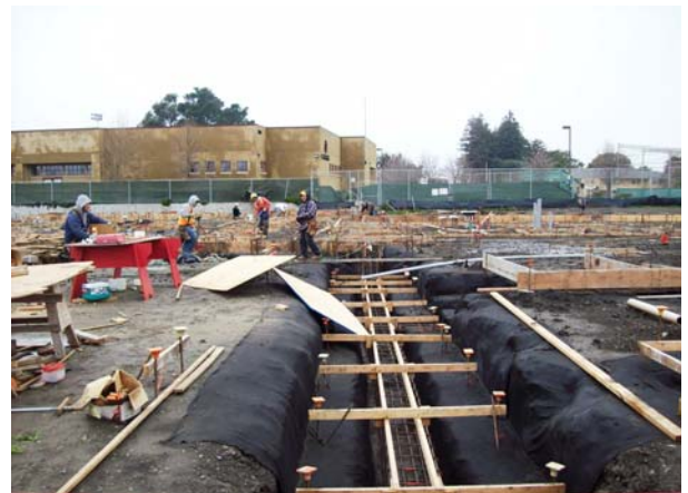
Areas B & C - Footing Development Continues
