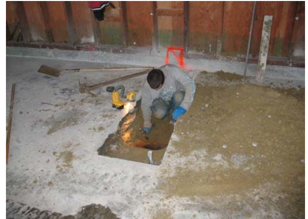
Locating sewer line
