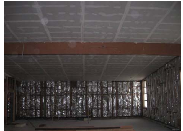
Insulation/Sheetrock Ceilings
