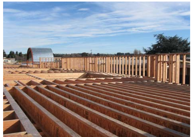
Installation of I-Joists & Parapets
