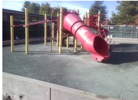
Valley View A @ Tot Play Yard Finish Grading
