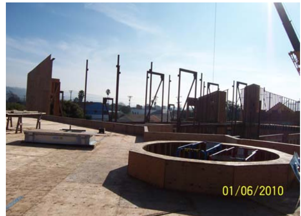
Building A: Waterproof Underlayment & Building Envelope
