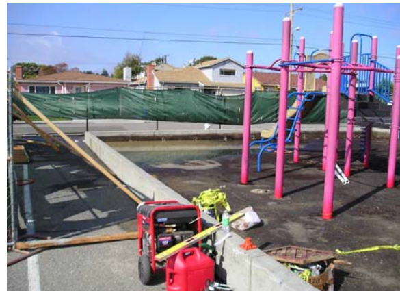
Wilson A - installation of Play Structure
