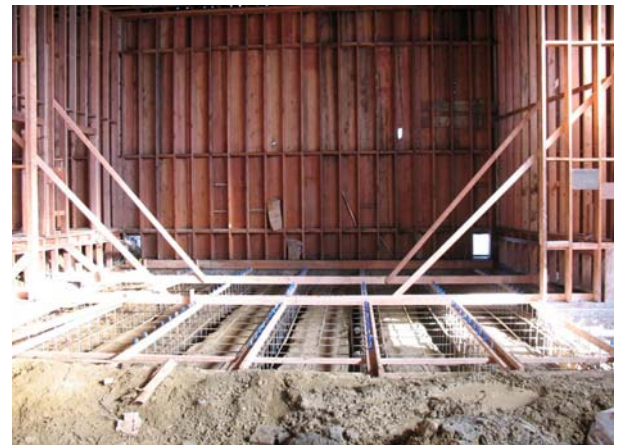
Ready to pour footings in Multi Purpose Room
