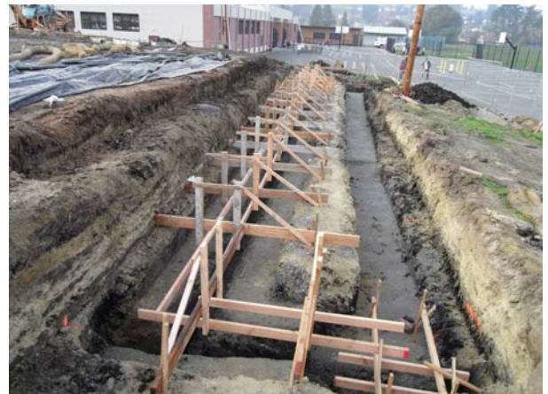
Construction of Baseball Field Retaining Wall Foundation
