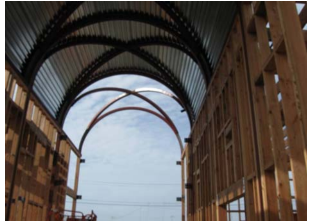
Interior Wall Framing & Steel Structure
