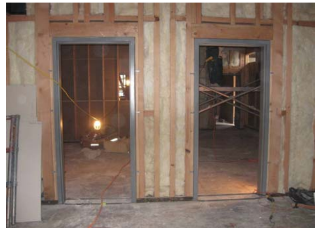
Interior Framing/Insulation/Door frames
