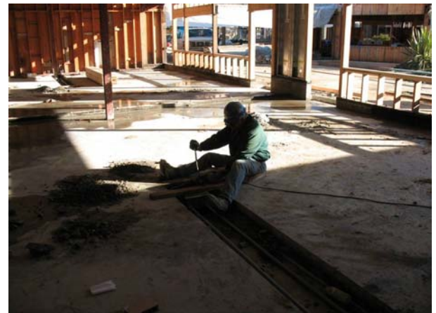
Drilling dowels into floor for conduit
