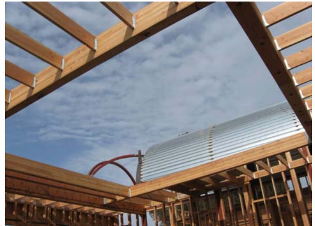
Installation of Roof Framing System & Skylights
