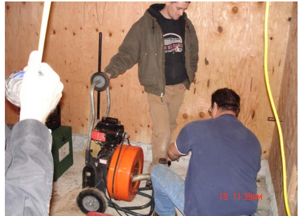
Sewer Line Probe - Bathroom 700-1
