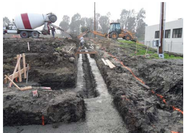
Construction of (N) Baseball Field Retaining Wall Foundation
