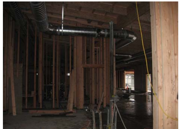
Duct Installation
