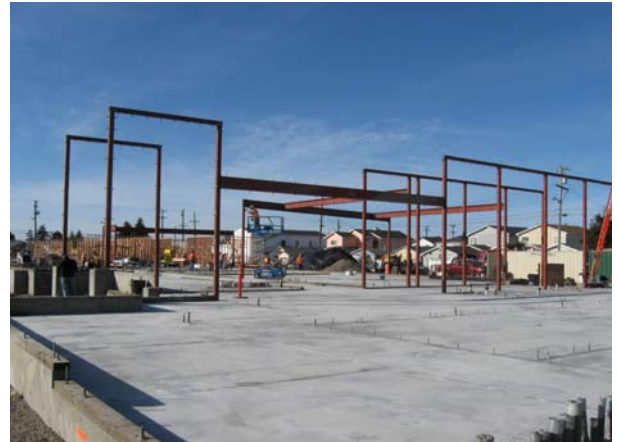
Erect Steel at North End of Building A
