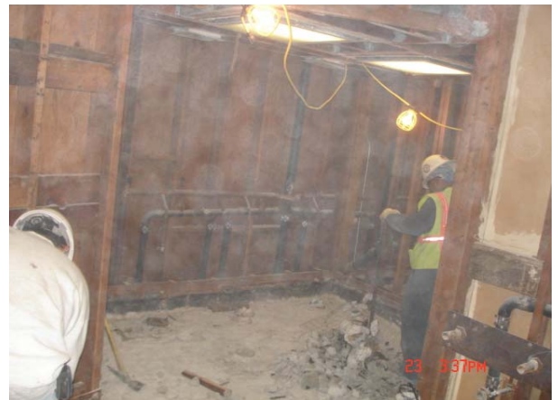
Work in Boy's Bldg. 200 Restroom
