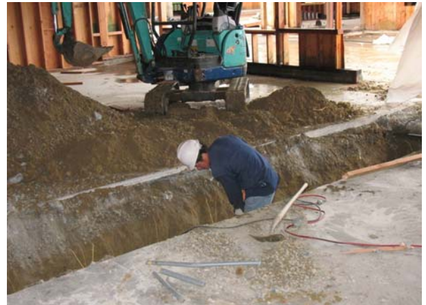
Excavating footing
