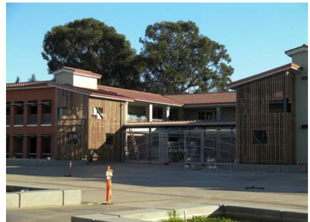
Bldg C: Gates and Cedar Trim @ Stairwells
