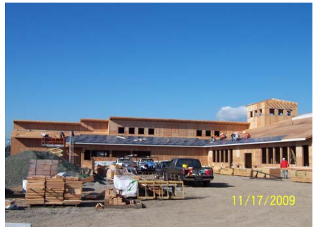
Building A West Roofing Underlayment
