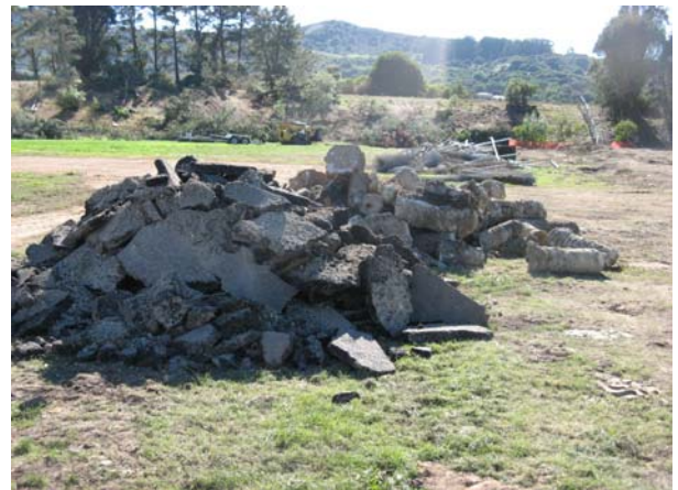
Demolition and Removal of (E) Baseball Field Infrastructure
