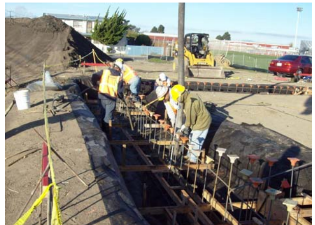
1st Concrete Placement Underway on 11/19/09
