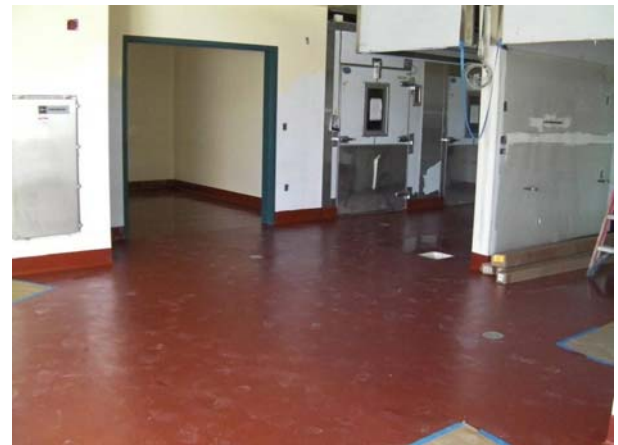
Kitchen Flooring: Installed
