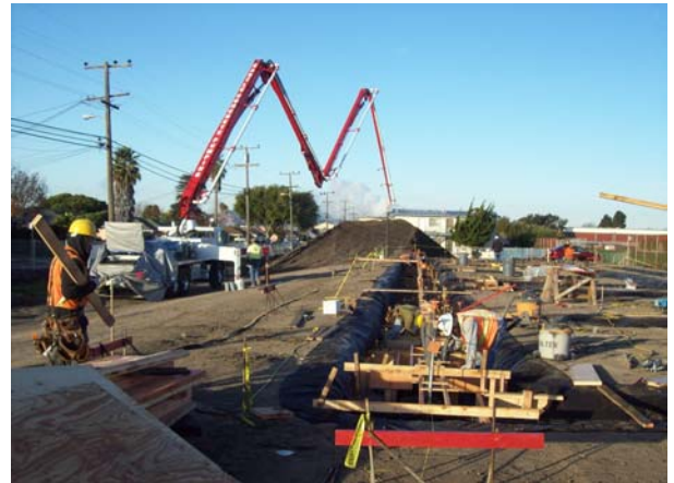
Set-Up & Ready for 1st Concrete Placement on 11/19/09
