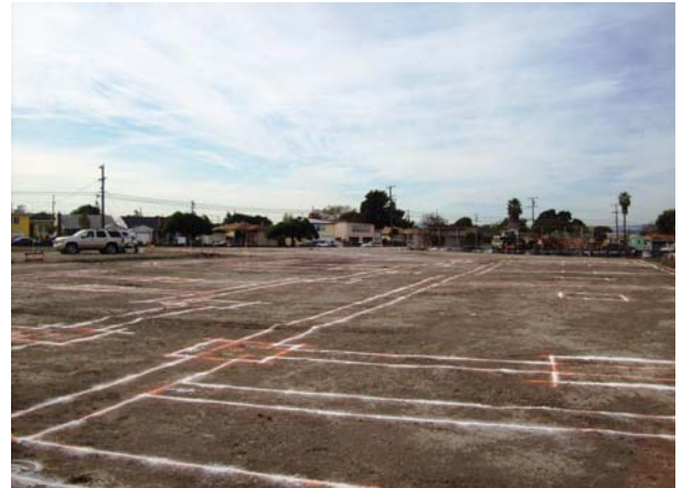
Layout Nears Completion on 11/9/09
