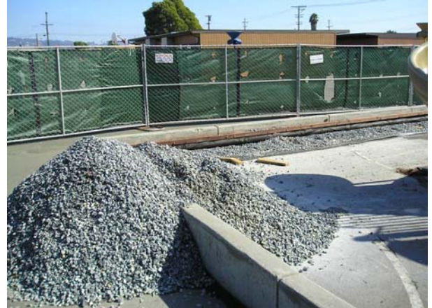
Coronado School Play Yard B - Drain rock placement
