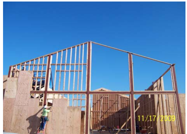
Building C Framing and Plywood Sheathing
