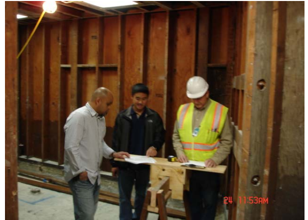
Construction Planning - Bldg. 200 Boy's Restroom
