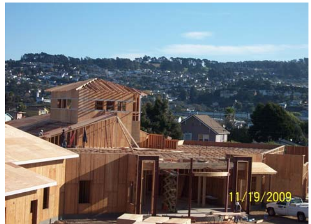
Building A East Roof Framing and Blocking
