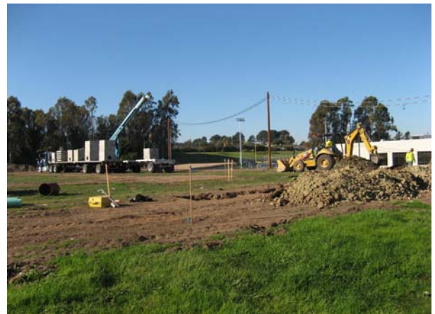
Installation of (N) Baseball Field Drainage Infrastructure
