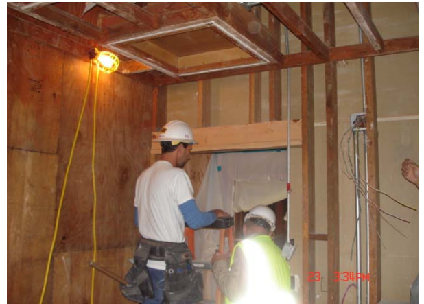
Work in Girl's Bldg. 200 Restroom
