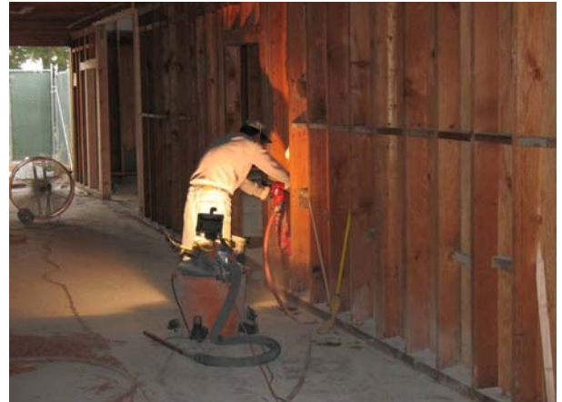
Drilling hold down bolts
