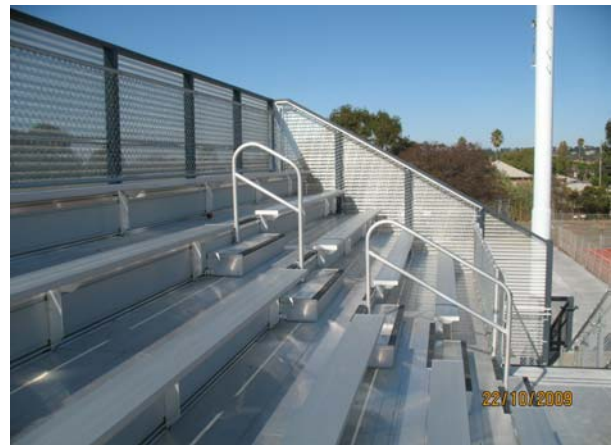
Detail view of bleacher seating and screening
