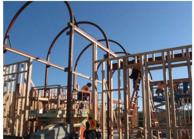
Exterior Framing at Building A Entrance
