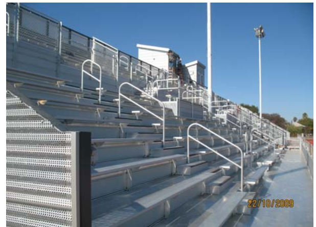
Bleacher seating, stairs and handrails complete
