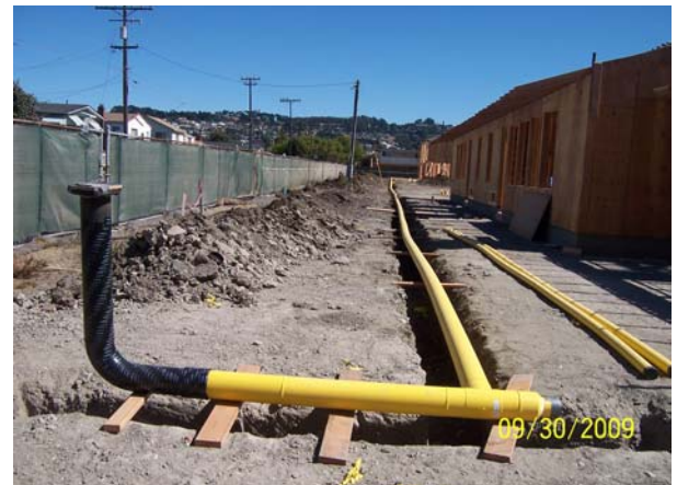
Gas Line at Building Perimeter
