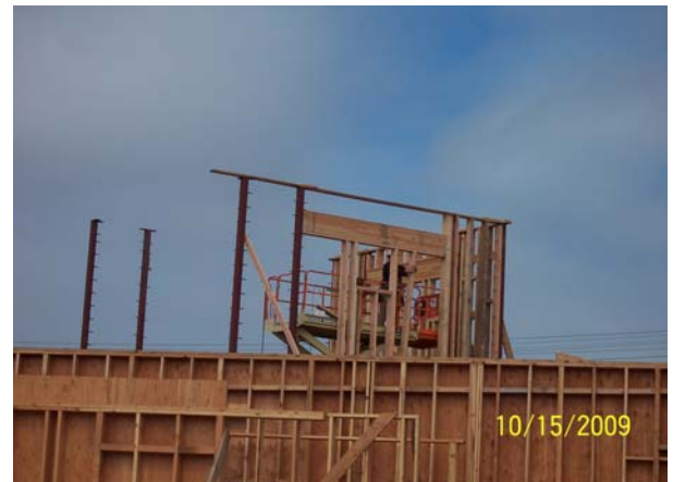
Tower Wall Framing and Shear Ply
