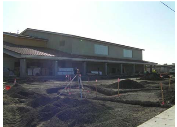
Visitor Parking Lot: Curbs poured & dug
