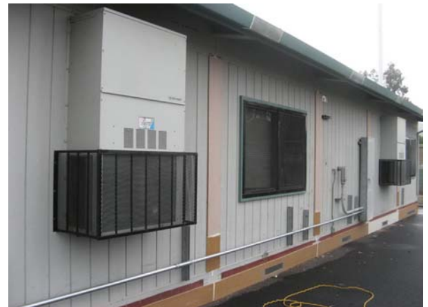
Installation (N) Protective Screens-COMPLETED
