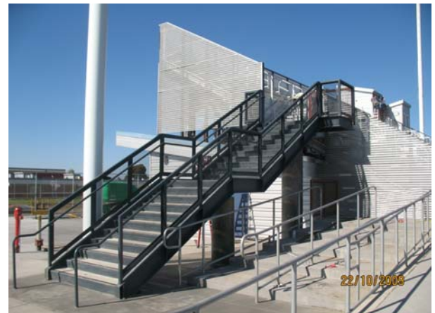
Main egress stairs poured and completed
