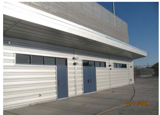
Completed exterior metal siding
