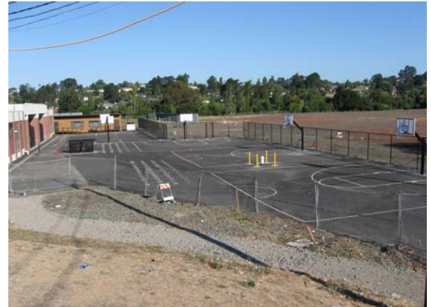
Application of Anti-Graffiti Application-COMPLETED
