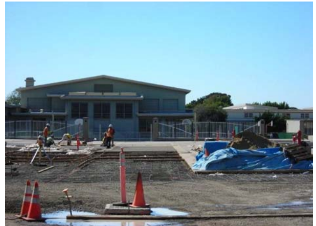
Main Courtyard: Concrete Walkways & Fence
