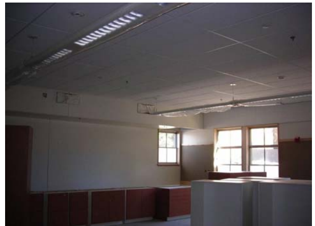
Bldg C1: Interior Finishes & Teaching Walls
