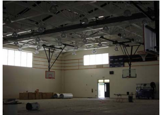
Bldg G: Lights, Divider, Basketball, Scoreboard
