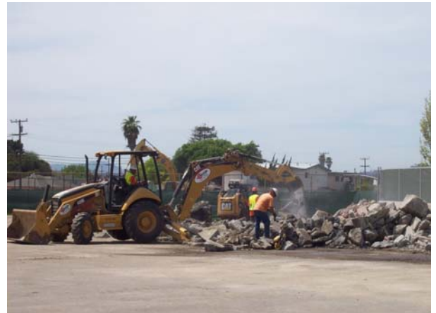
AC & Base Removal
