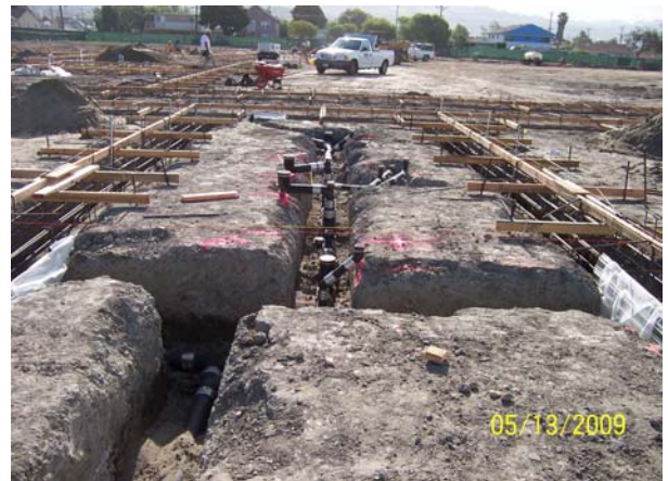
Underground waste and electrical rough-in
