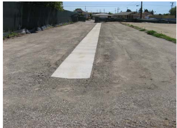
Increment 1A-Concrete Swale and Parking Area-COMPLETED
