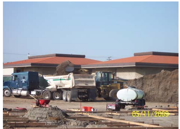
Off-haul of excavation spoils
