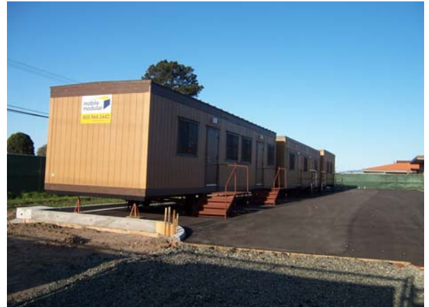
Construction Trailer Delivery & Set-up
