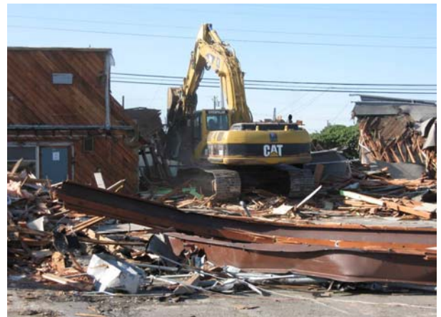
Existing Building Demolition
