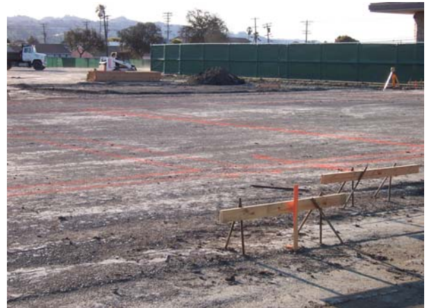
Site Survey and Footing Layout
