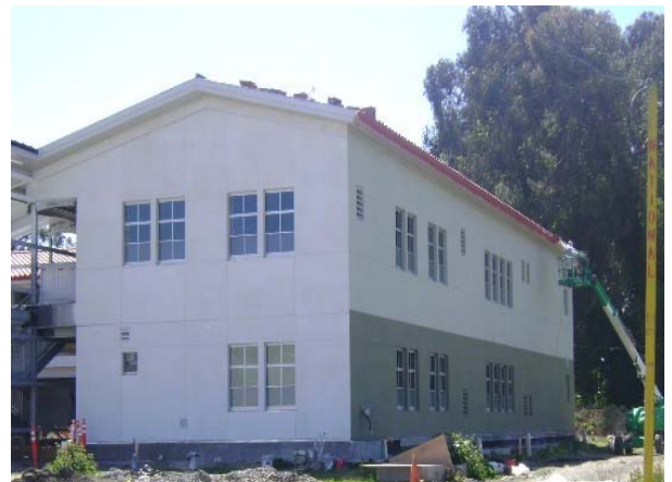
Building C3: Exterior Painted Stucco Finish
