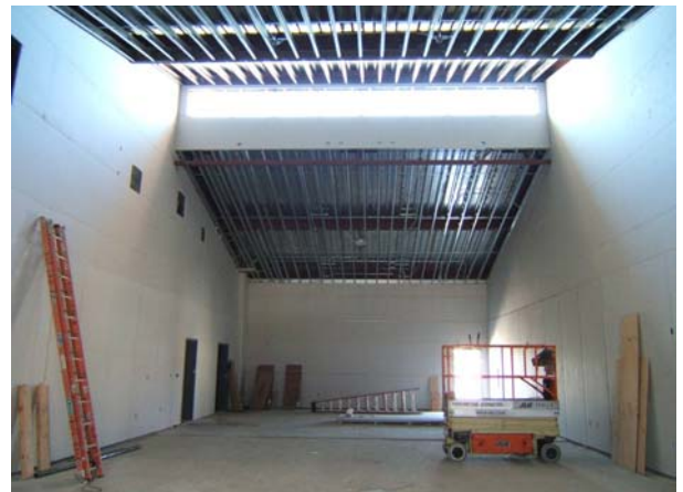
Building G: Interior Gyp & Clerestory Window
