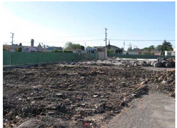
Footing and Foundation Removal
