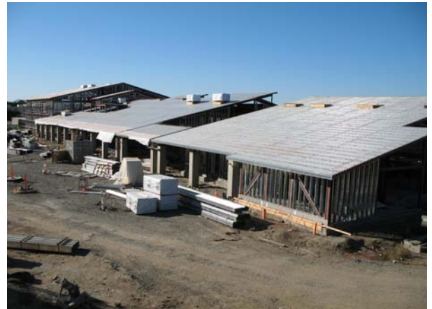
Framing & Roof-Plywood & Sheathing @ Bldg. G, MCA
