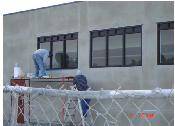
Installing Window Trim
