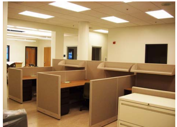
Health Clinic Offices Essentially Complete
