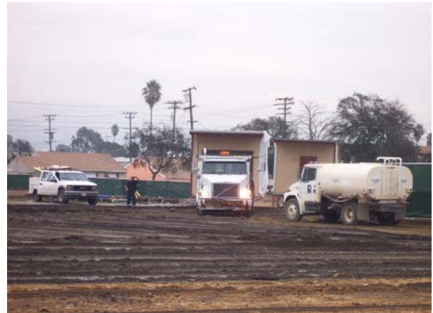
Relocation of Portable Building
