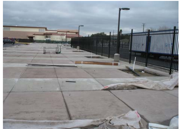
Completion of Concrete Paving and Installation of Fencing
