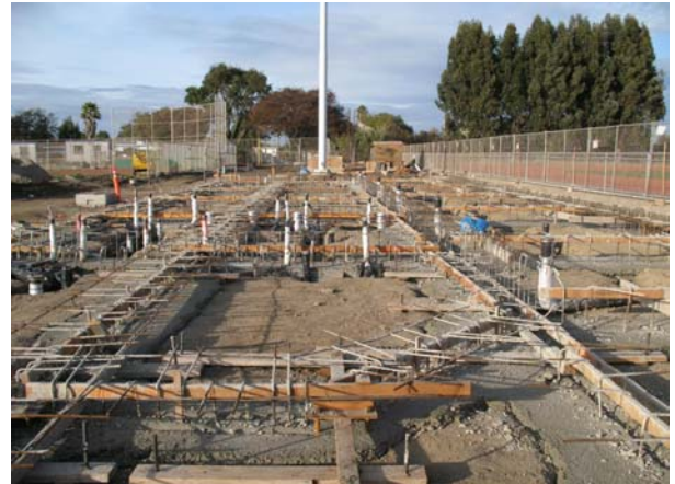
All concrete footing are poured and ready for steel
