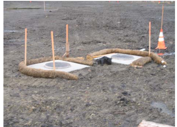
Storm Drain Installation
