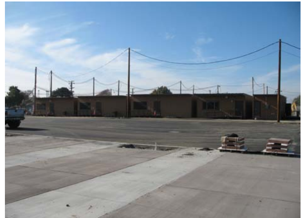
Installation of Asphalt and Concrete Pavement
