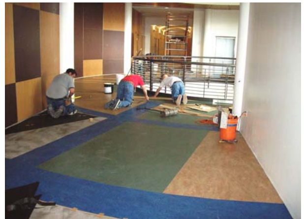
2nd Floor Rotunda Balcony Nears Completion
