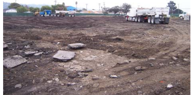
Demolition & Removal of AC and Rough Grading
