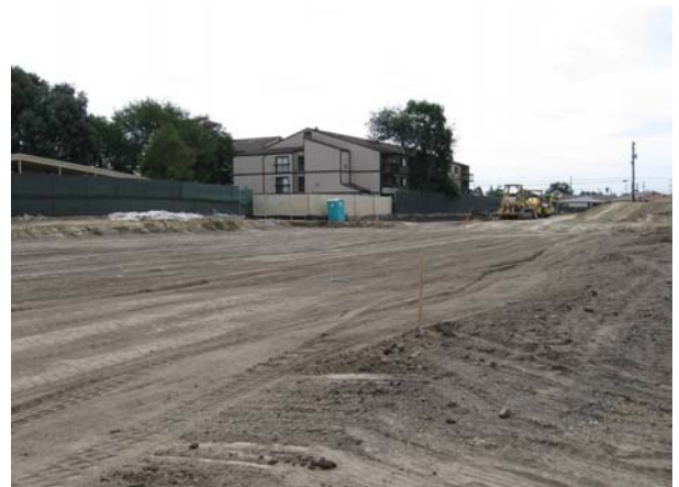
Site Rough Grading
