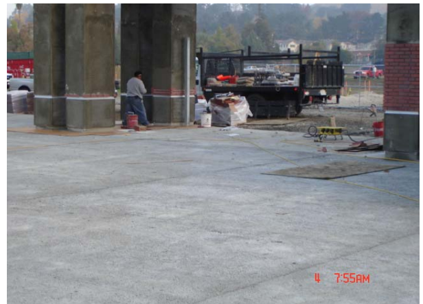
Brick Installation on Columns
