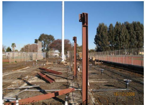
Structural steel columns installed
