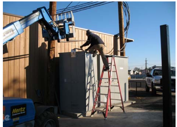
Installation of Electrical and HVAC Infrastructure
