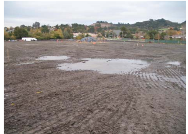
Site Rough Grading
