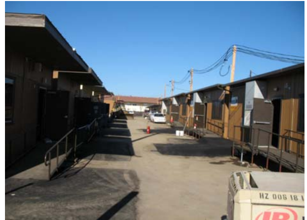
Installation of Modular Units
