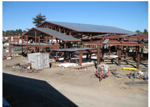
Metal Roof Decking @ Bldg. M
