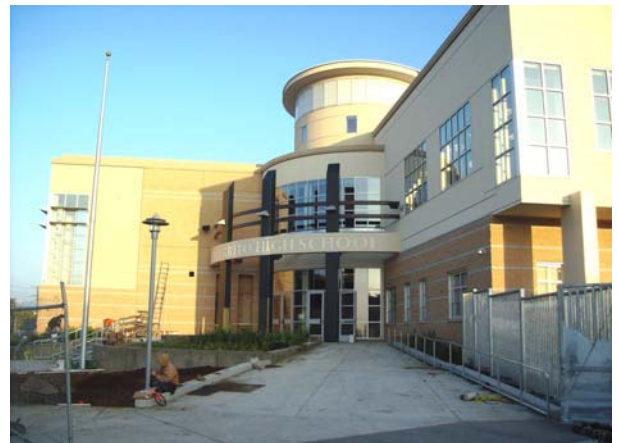
Main Entry to Rotunda Lobby Nears Completion
