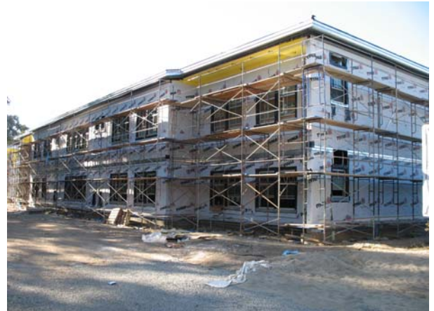
Exterior Drywall & Window Installation @ C1, C2.
