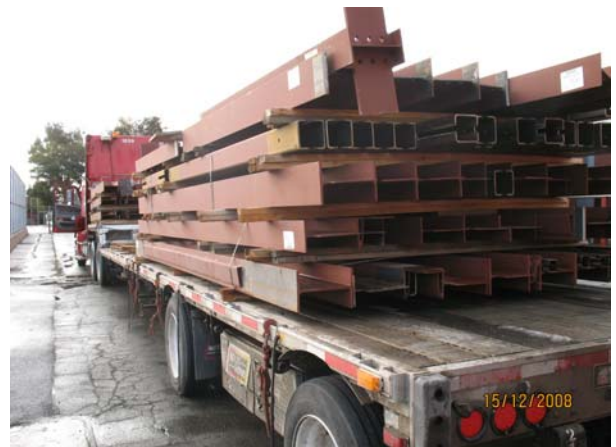
First structural steel delivery
