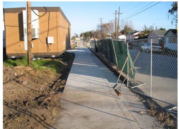
Completion of Sidewalk Installation
