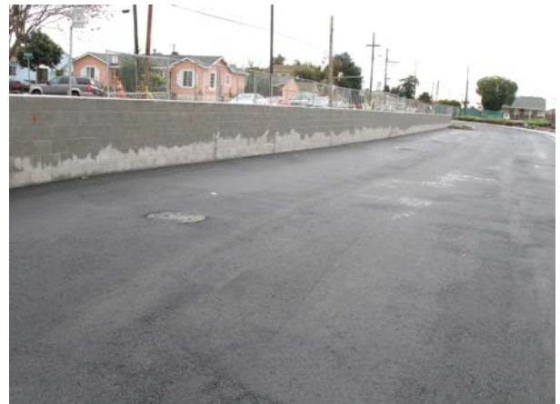
Completion of CMU Wall and Asphalt Parking Lot
