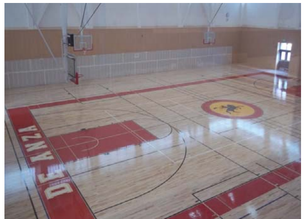
Building 8--Main Gym Floor Installation & Striping
