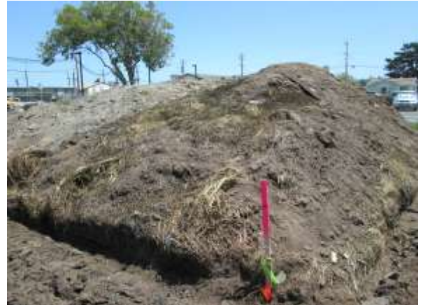
Existing soil with vegetation and waste debris
