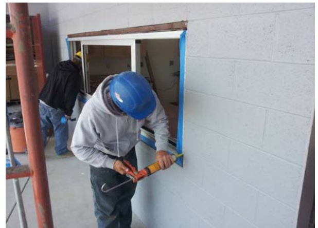
Concession Stand - Serving Window Installation
