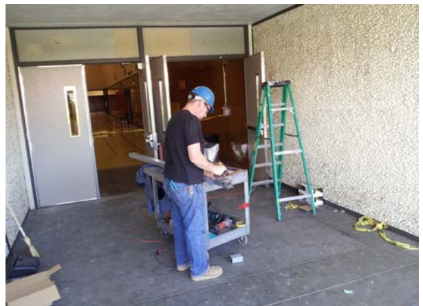
Gym Door Installation
