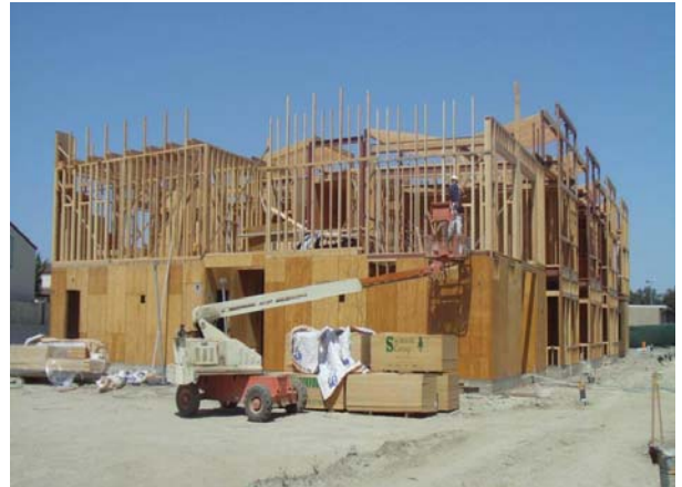
Building A First and Second Level Rough Framing
