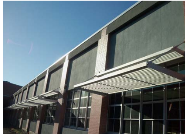
Building 6--Sunshade Installation
