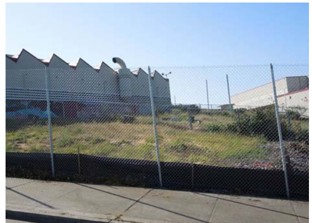
Initial SWPPP Installations are Progressing
