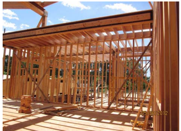
Building A Second Story Classroom Framing
