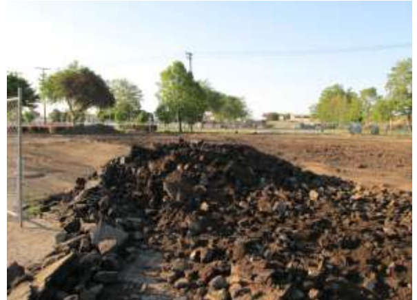
Site Grading and asphalt demo work
