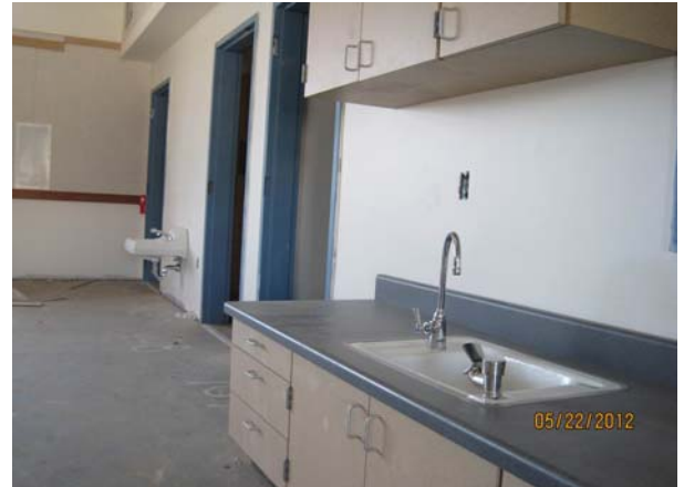
Bldg B Finishes - Casework, Fixtures, Trim
