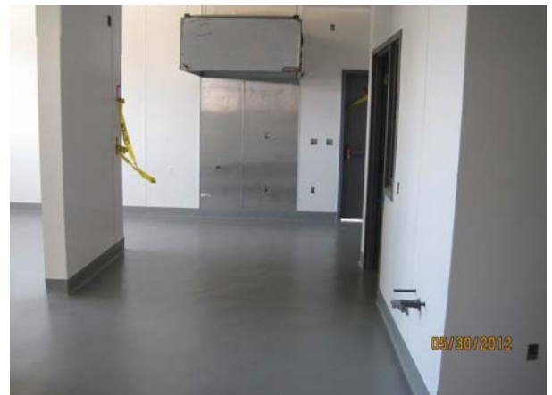
Bldg C Finishes - Urethane Flooring, Hood, FRP
