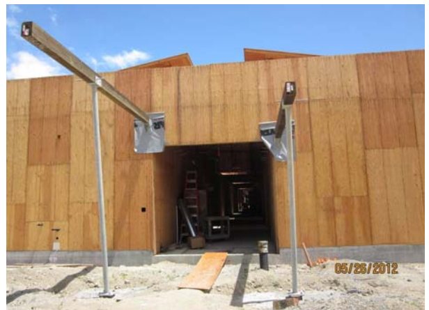
Building B Canopy Framing At West Hallway Entrance
