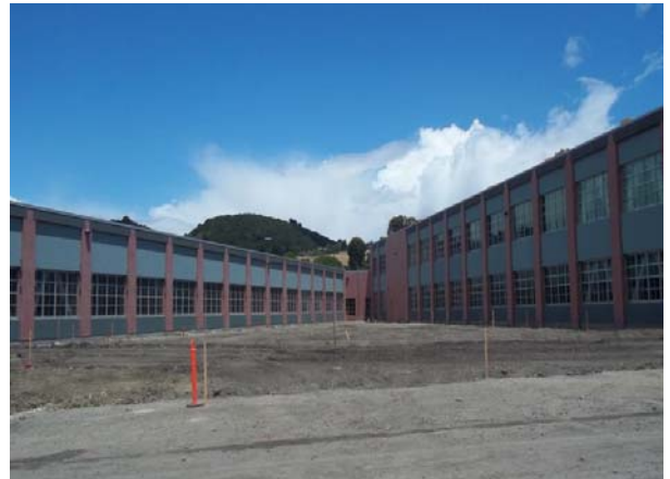
Building 7--Rough Grading for Courtyards
