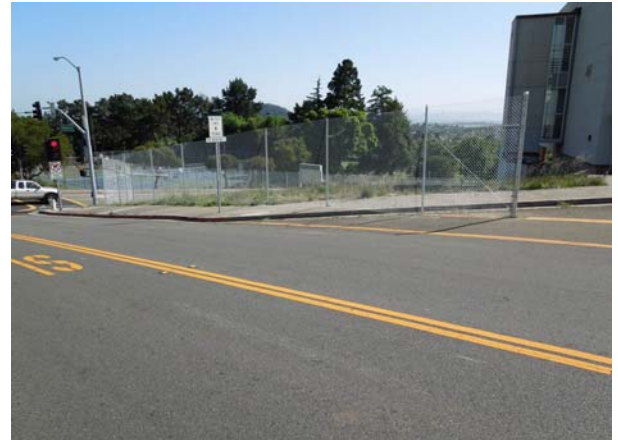
Perimeter Construction Fence Installation Underway
