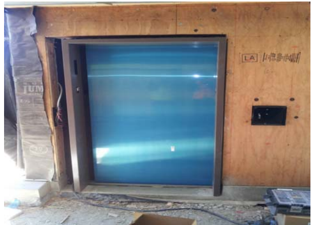
Installed Elevator Door
