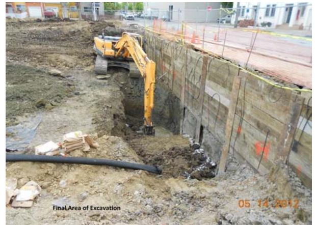
Final Area of Excavation
