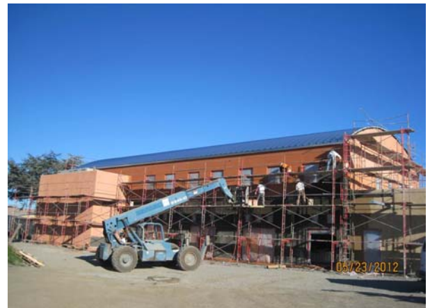
Building C - Plastering - Color Coat
